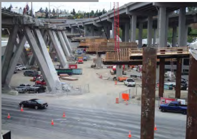
Crews are building a bridge (center piers with wood forming) that will temporarily carry eastbound SR 16 traffic while the original eastbound Nalley Valley viaduct (on left) is demolished and rebuilt.
