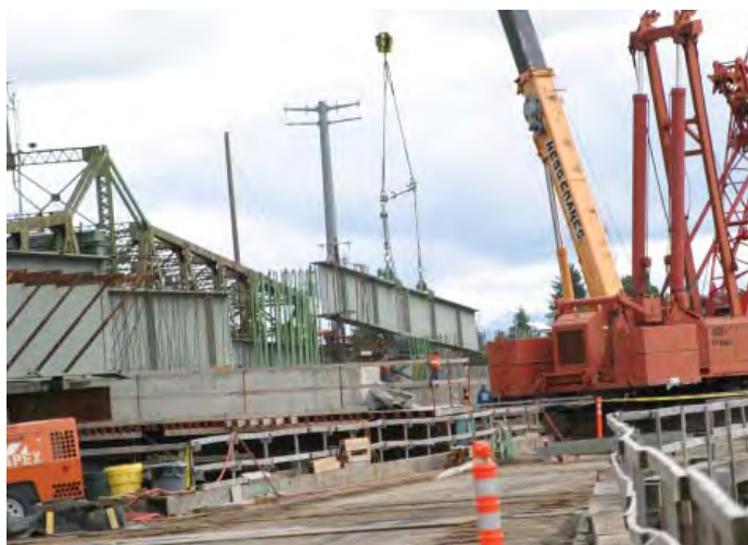
A crane lifts a girder section into place at SR 529 Ebey Slough Bridge.
