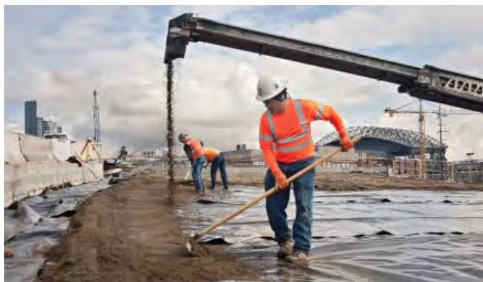
Crews spread sand on the south approach to the northbound SR 99 bridge under construction.
