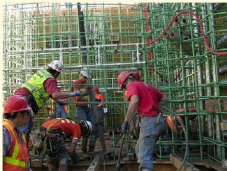
Workers spread concrete and work it down between rebar and conduit in the first pontoon concrete pour April 28, 2006.
