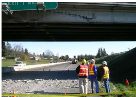
Crews began repairing damage to the SR 14 Lieser Road Bridge in May. An oversize load hit the bridge in November 2005.
