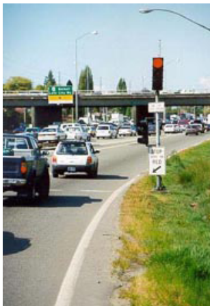
A ramp meter controls the flow of traffic onto the highway, increasing average speeds on the road.
