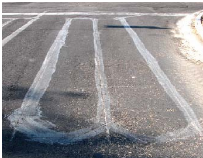
An induction loop embedded in the highway collects traffic data and sends it to a traffic management center.
