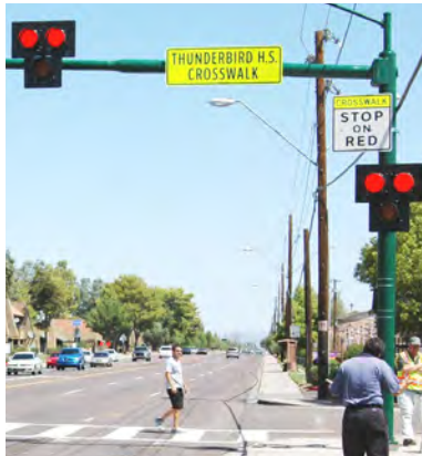
A push-button activated pedestrian hybrid beacon signals drivers to stop on red for pedestrians to cross the street. Source: www.pedbikeimages.org/ / Mike Cynecki
