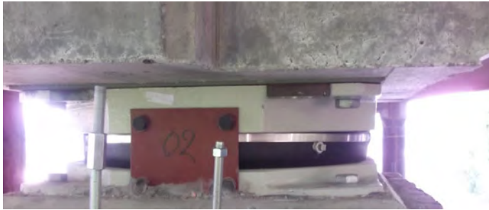
Two slabs of concrete separated by a 2-foot, 7-inch diameter bearing are what stands between Aurora Bridge drivers and disaster in an earthquake. This huge bearing allows the bridge to sway any direction with a tolerance of 1-foot. Massana Construction installed these bearings in October 2012.
