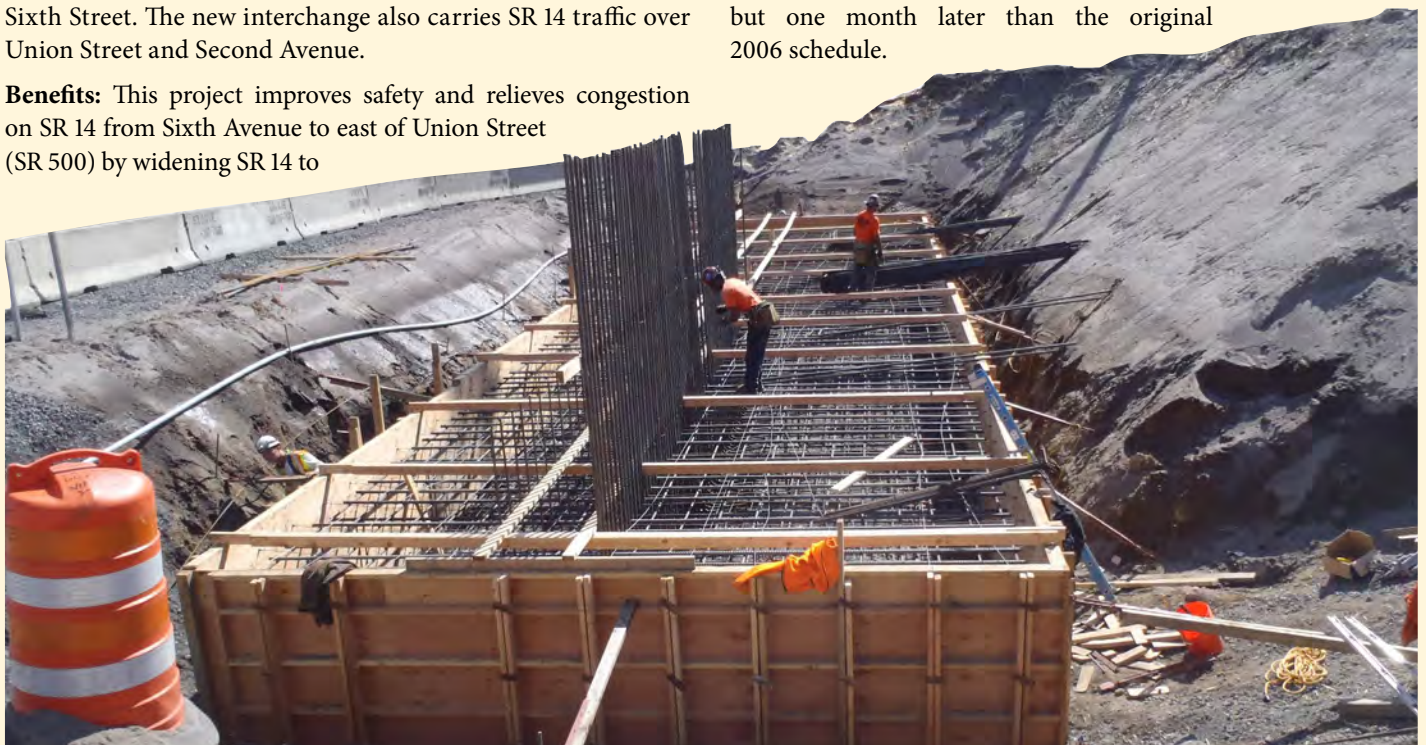
Crews construct footings to support the new Union Street Bridge in March 2012. The SR 14 project built a new interchange to carry traffic over Union Street and Second Avenue, relieving congestion between Camas and Washougal.
