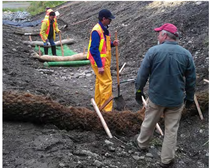
Students of the Certified Erosion and Sediment Control Lead certification program install erosion control mats and check dams, which is a best management practice to control stormwater runoff.
