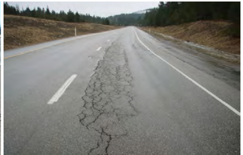
Asphalt pavement in very poor condition: past due for rehabilitation, will require costly repair.
