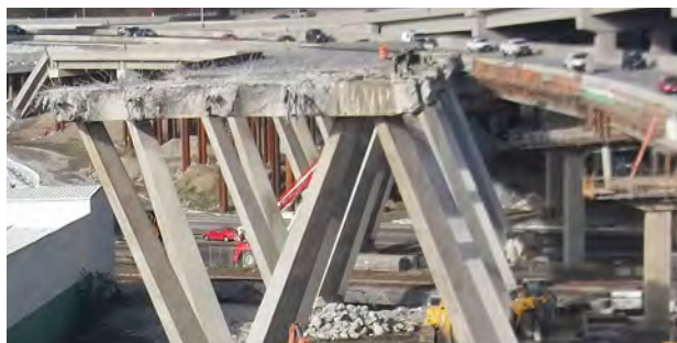
This is a view of the original SR 16 Eastbound Nalley Valley viaduct's unique tetrapod support structure. Demolition is expected to last through March 2013.
