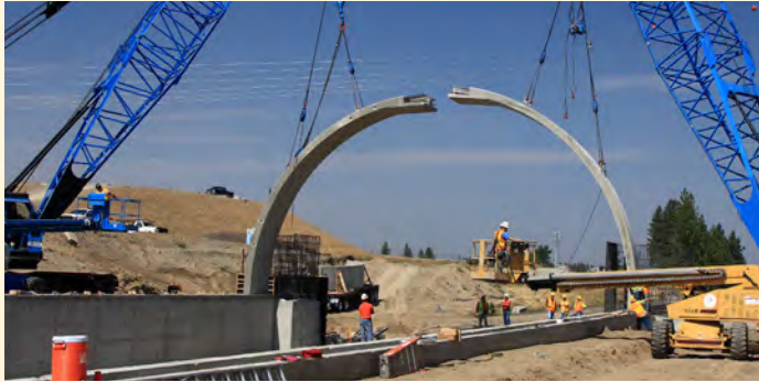
A new tunnel to accommodate BNSF trains is just one of the projects included in North Spokane Corridor work completed to date. Here cranes lift 42,000-pound sections into place to form the tunnel's arch.
