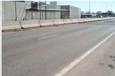
Asphalt pavement in fair condition: wear in wheelpath and transverse crack across the road.
