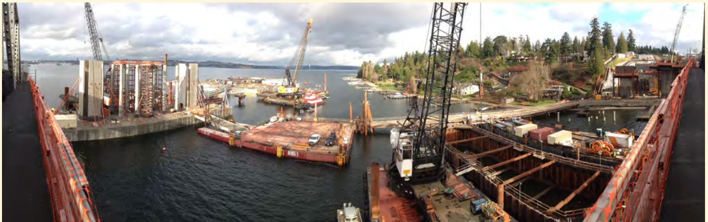
A panoramic view of the SR 520 bridge work from the East Approach area near Medina. Box columns are constructed on Pontoon W (center left) as water is pumped out of a cofferdam (below right), which will allow crews to safely work nearly 40 feet below the surface of Lake Washington.
