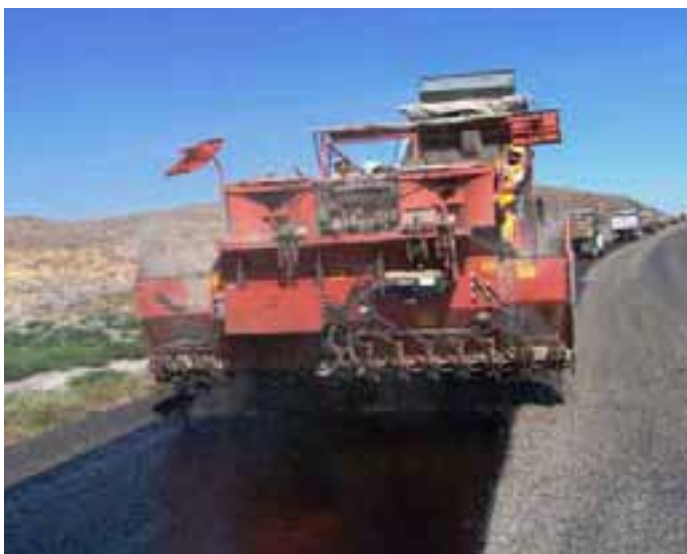
Applying the "oil" (polymers) and "chips" (gravel) during a chip seal paving project in the North Central Region.
