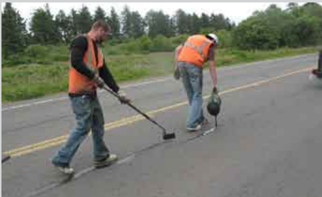
Crews seal cracks in asphalt to prepare for chip sealing on SR 103.
