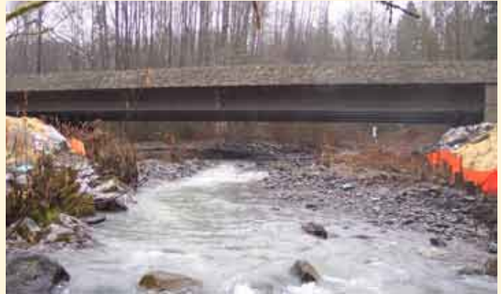
This project built a new bridge over Gallup Creek and realigned SR 542 and redirected the Nooksack River to address rising flood risk that endangered washing away the road.
