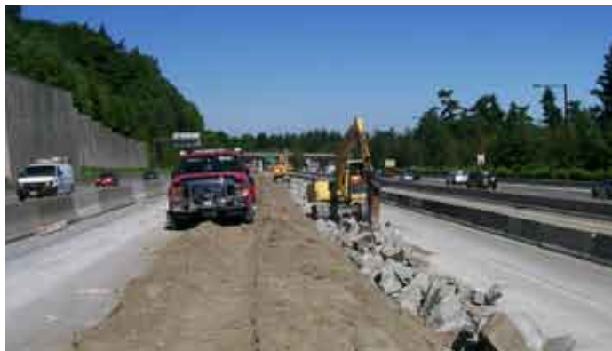
Stage 2 of the I-90 Two-Way Transit and HOV project was under construction in August 2010. In order to widen the roadway crews must demolish the existing barrier. This is the view looking west. The center roadway and westbound I-90 are on the right.
