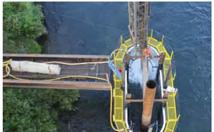
A "bubble curtain" is sometimes used to lessen the sound caused by driving piles for construction piers and/or building facilities that are located over water.
