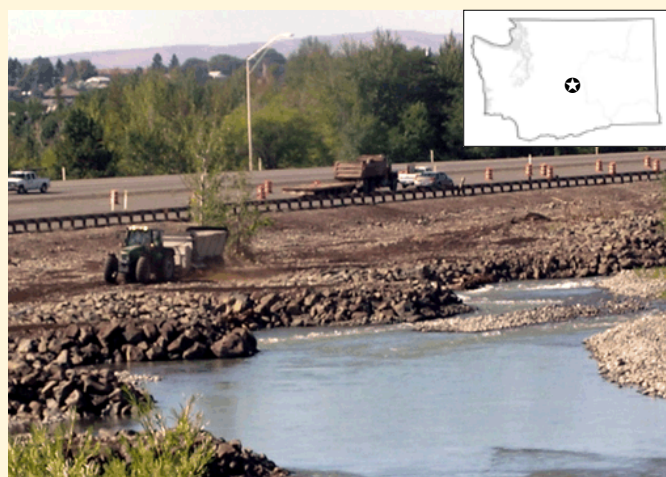
The Naches River slope stabilization at US 12 helps protect the highway from erosion.
