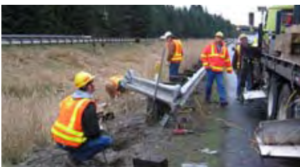
Maintenance crew repairs a damaged guardrail.
