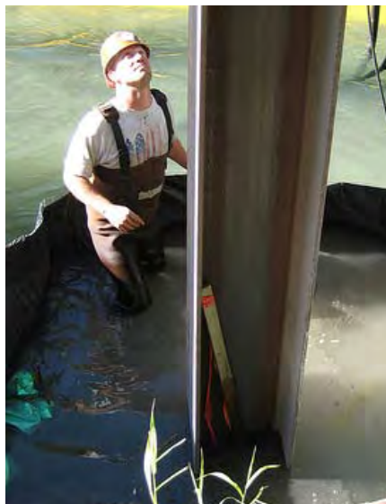
A worker guides a steel piling for the log wall into place on the Sauk River.
