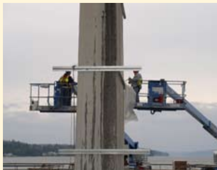
Crews saw cut the old approach span pier into sections for removal.
