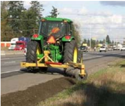
A WSDOT employee performing annual cultivation. This helps maintain a vegetation free zone at the edge of the pavement without the use of herbicide.
