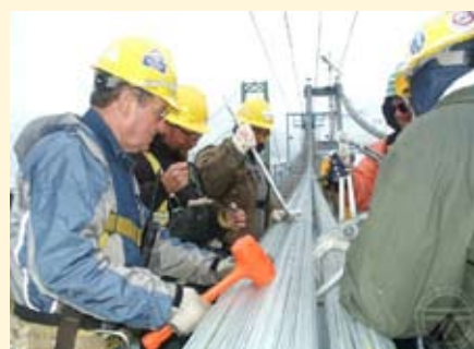
Compacting and banding strands on the north cable.
