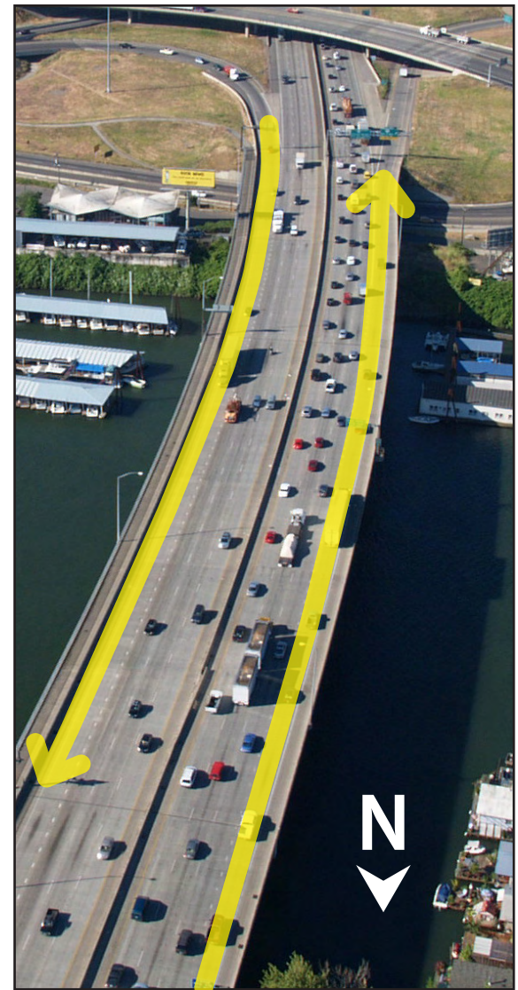
Auxiliary lanes between Hayden Island and Marine Drive.
