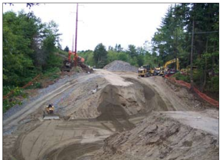
Replacing the culvert required cutting out a section of the highway.
