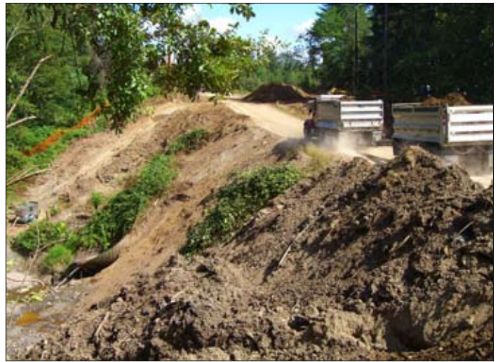
The culvert was 25 to 30 feet below the road, making it difficult to get to.
