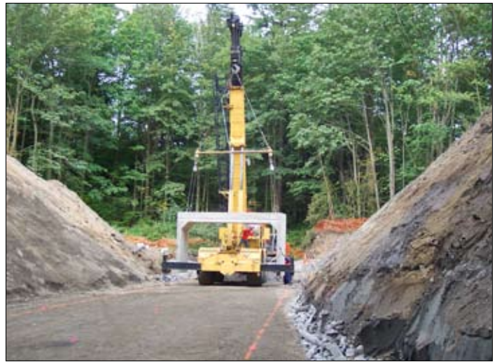
A crane lowers one of the first sections of the culvert into place.
