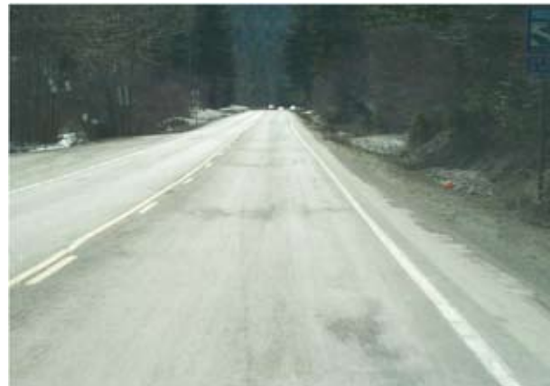
Figure 2. Cyclic pattern of low-density, permeable areas.
