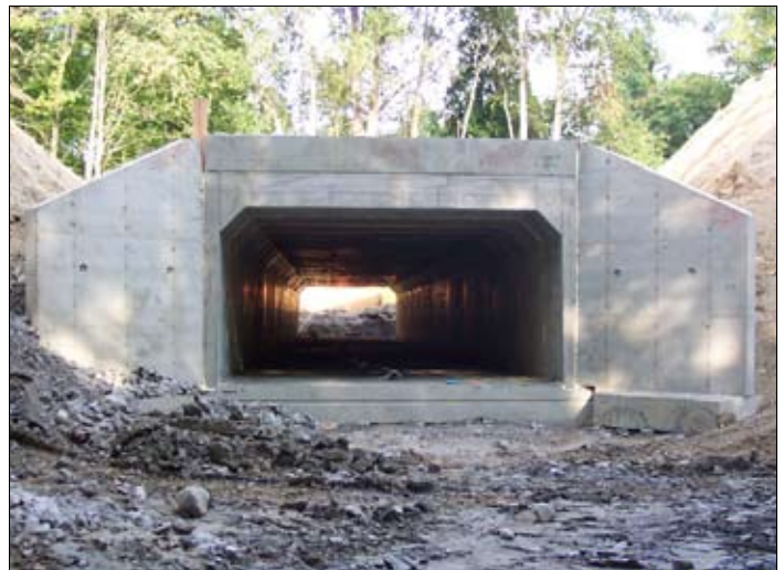
The new culvert measures 145 feet long, 18 feet wide, and 10 feet tall.
