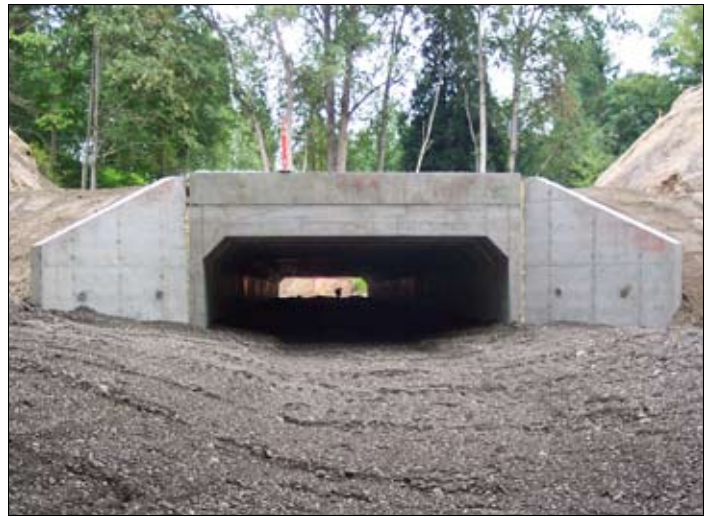
Crews laid streambed gravel across the base of the new culvert creating a seamless transition with the natural streambed.
