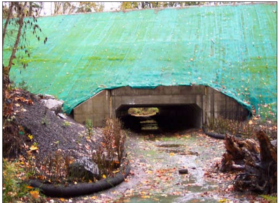
Water starts flowing through the new culvert.
