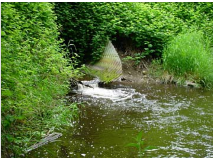
The broken ends of an old steel culvert flipped up when water was running high, blocking passage for fish trying to swim upstream. The broken culvert also was an indication that water could be seeping in around the pipe, jeopardizing the road above.
