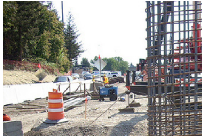
I-205 and 112th pouring concrete footings
