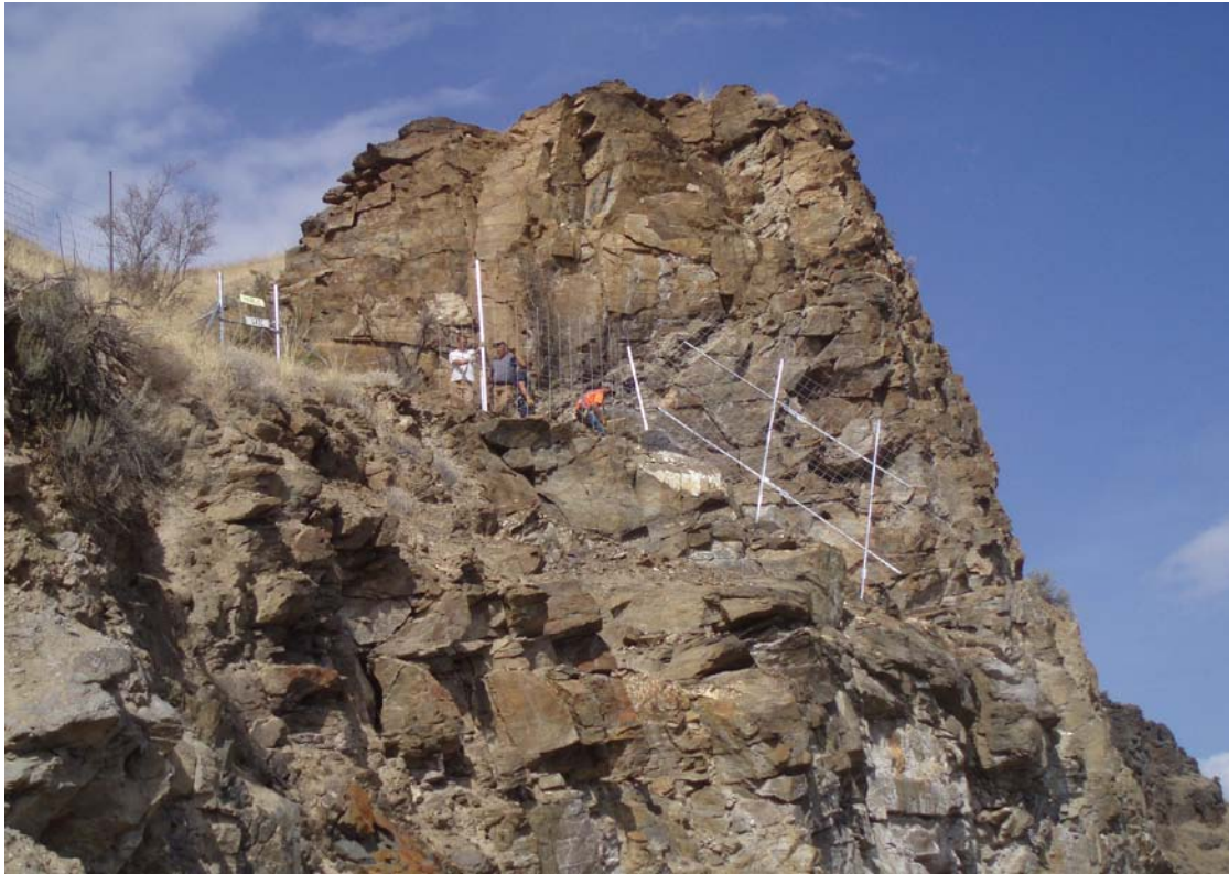
Installing Wildlife Fencing
