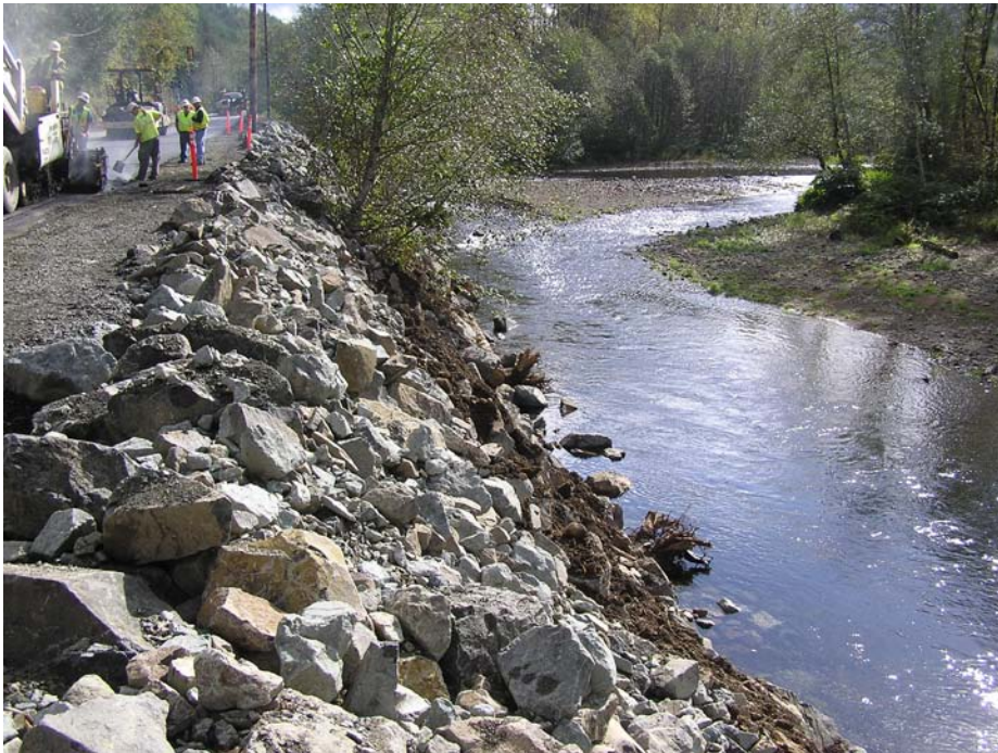
Rock Revetment and Large Woody Debris
