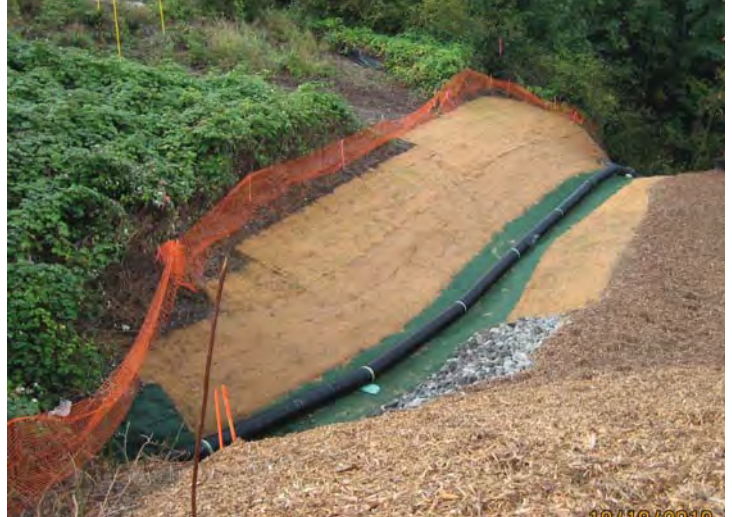
Figure 2: View of stream mitigation site.
