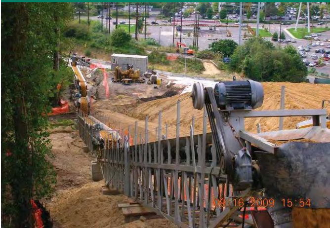
Figure 6. Conveyor kept pace with fill, keeping excess embankment onsite.
