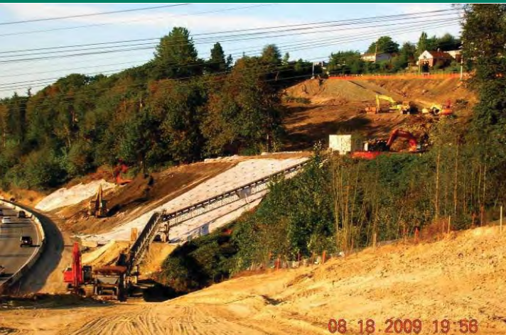
Figure 5: Conveyor system obviated 10,000 truck trips through the City of Renton.
