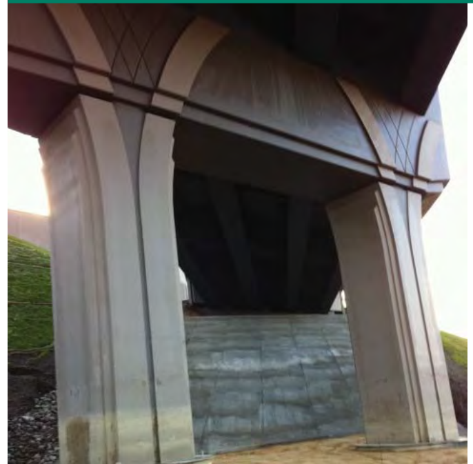
Figure 4: Benson Road Bridge showing the CSS aesthetic treatment.
