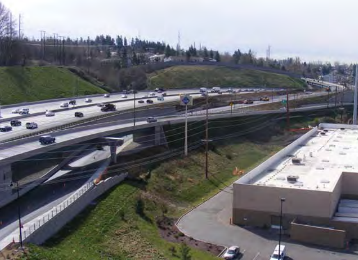
Figure 1: View of completed project.
