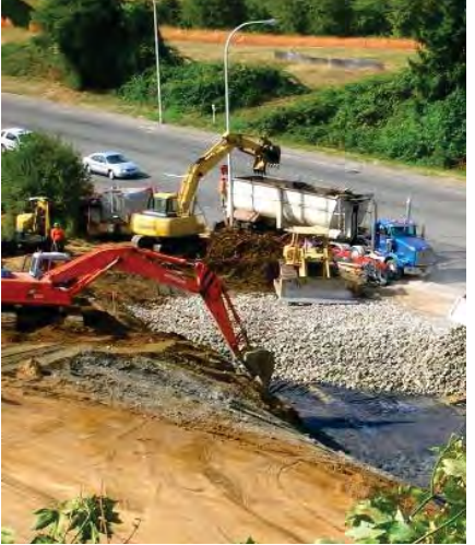
Figure 19. Lower cell placed over separation fabric. Quarry spalls filtration system.
