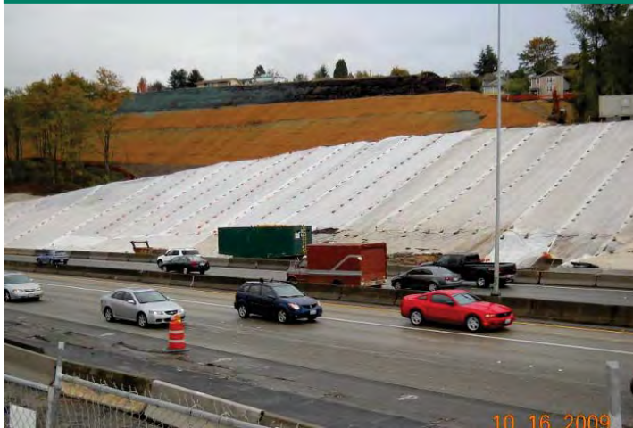
Figure 13. Permanent fill slope covering was installed as fill slope was constructed.
