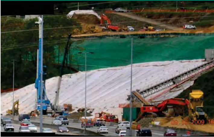
Figure 11. Permanent fill slope covering was installed as fill slope was constructed.
