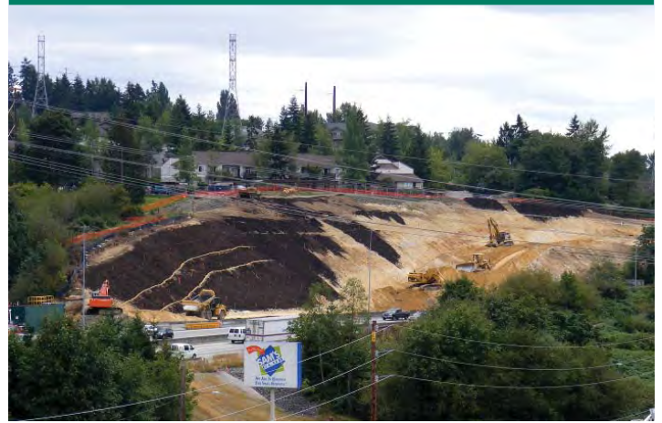
Figure 10. Permanent slope covering was installed as excavation proceeded.
