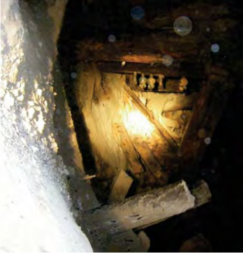
Figure 18. Diversion well casing, cut-off wall, and observation casing at abandoned mine shaft.
