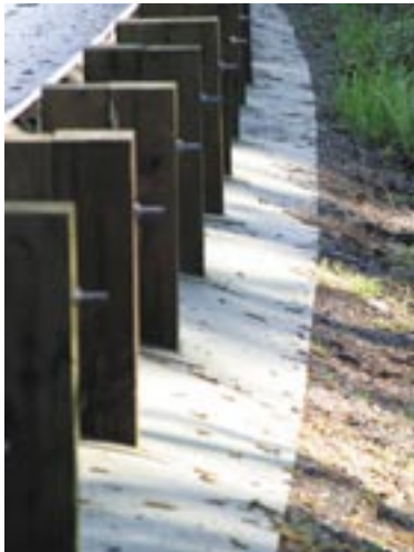
The pictured product is a mat that is installed underneath runs of guardrail and fits tightly around the base of guardrail posts. The mat prevents vegetation growth without the use of herbicides or labor-intensive trimming.
