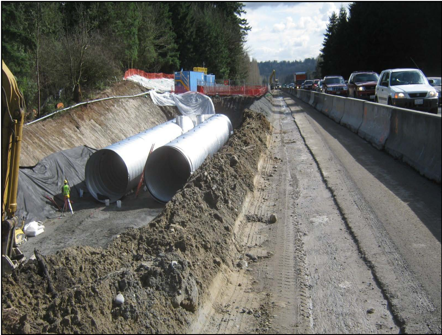
Kiewit crews begin installation of two underground detention vaults.
