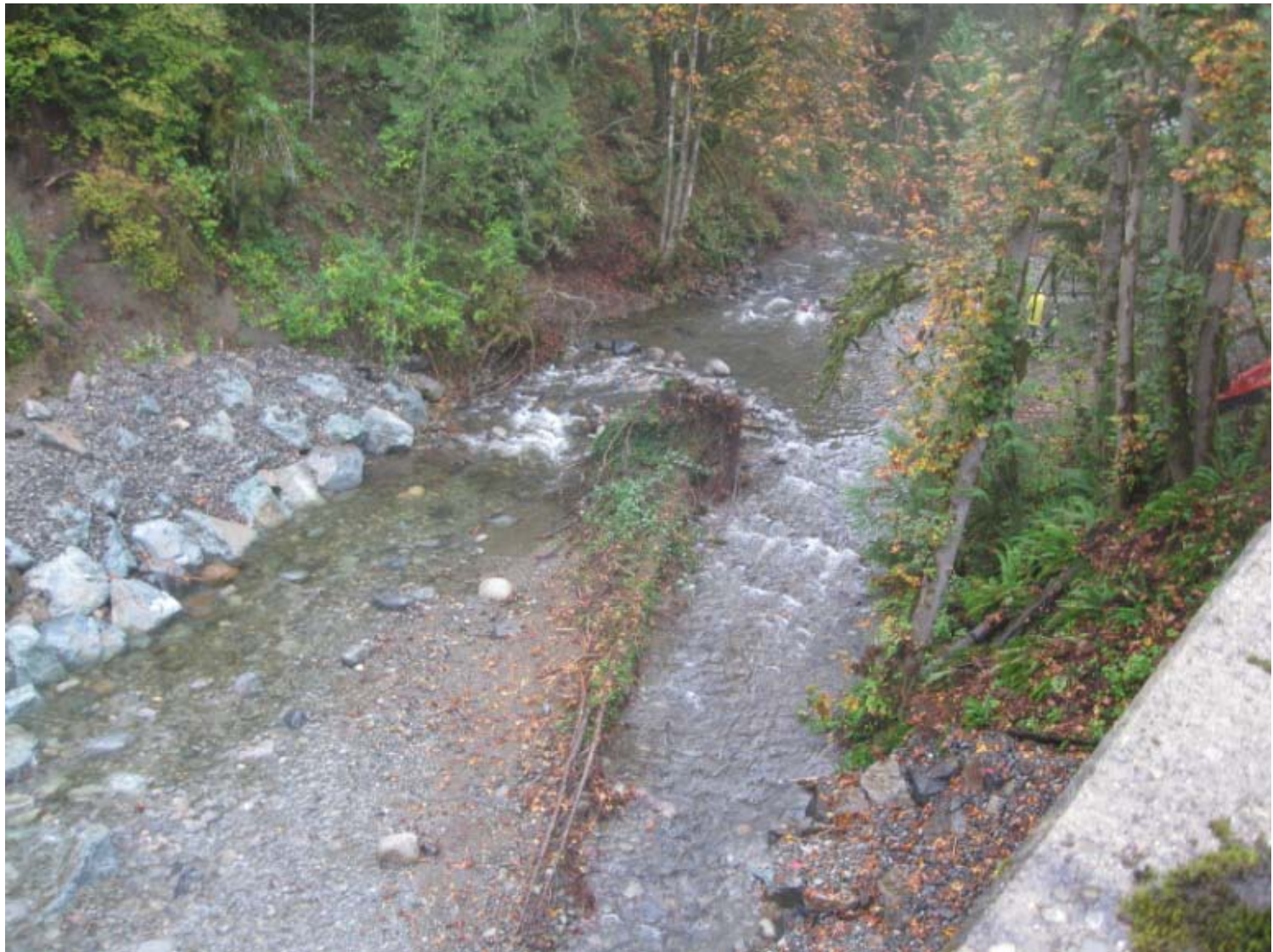
The restored creek, north of the Tokul Creek Bridge...
