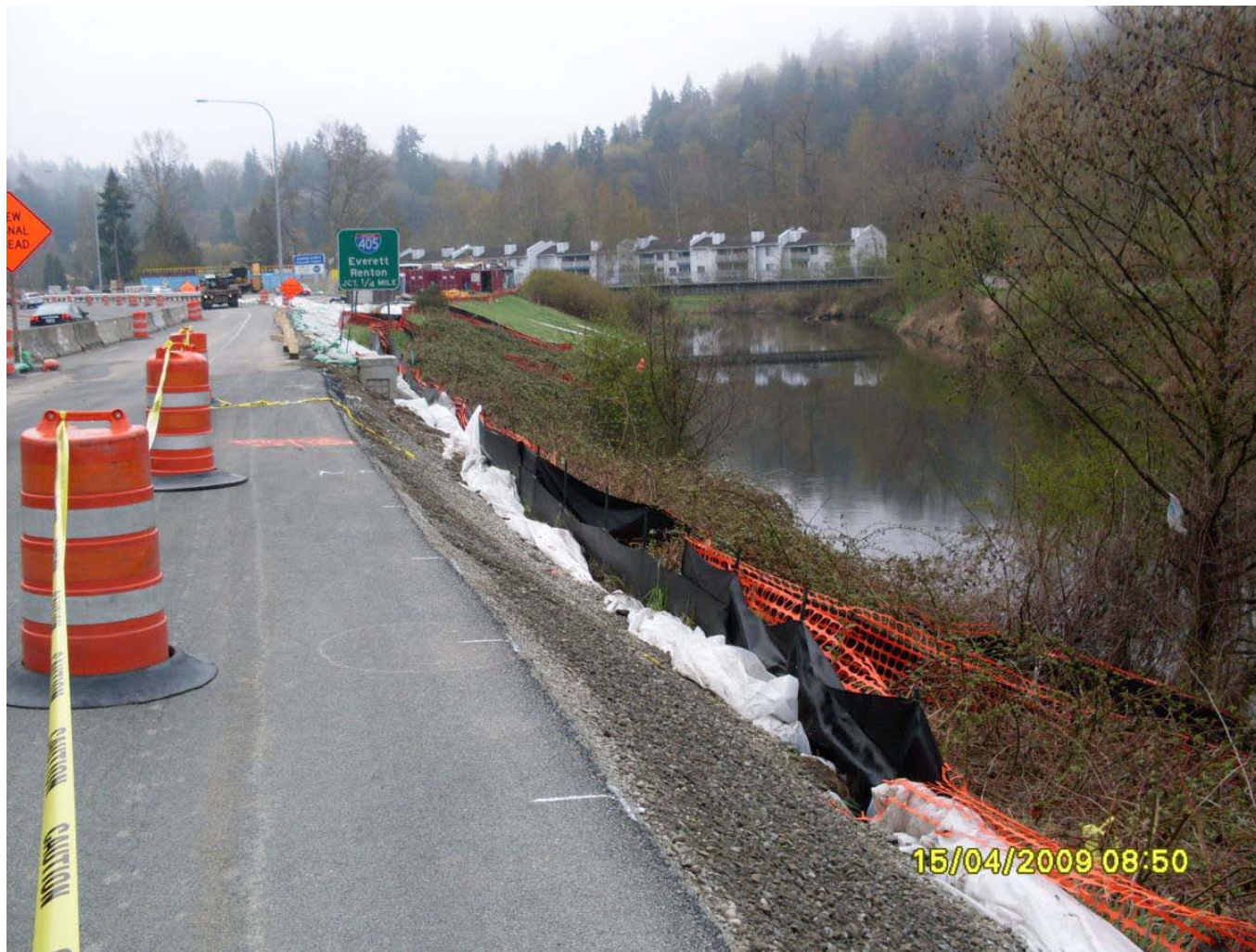
Roadway widening adjacent to the Sammamish River
