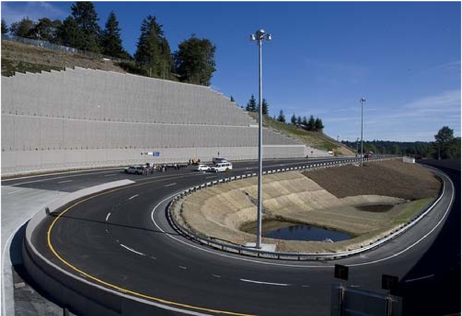
Wall and stormwater treatment pond at entrance to the UW Bothell / Cascadia Community College.
