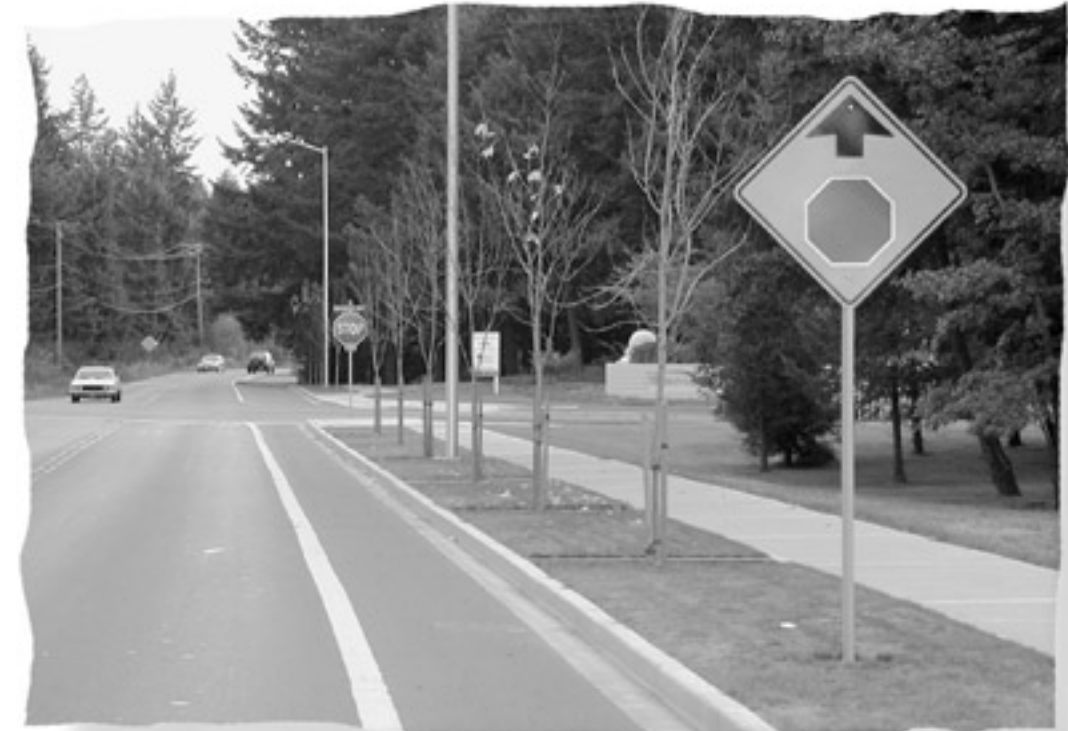
Figure 2. A properly installed Stop Ahead (W3-1a) sign.
