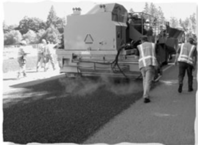
Live bottom truck supplying rock and emulsion.
