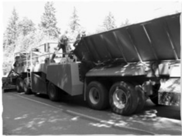
Live bottom truck supplying rock and emulsion.
