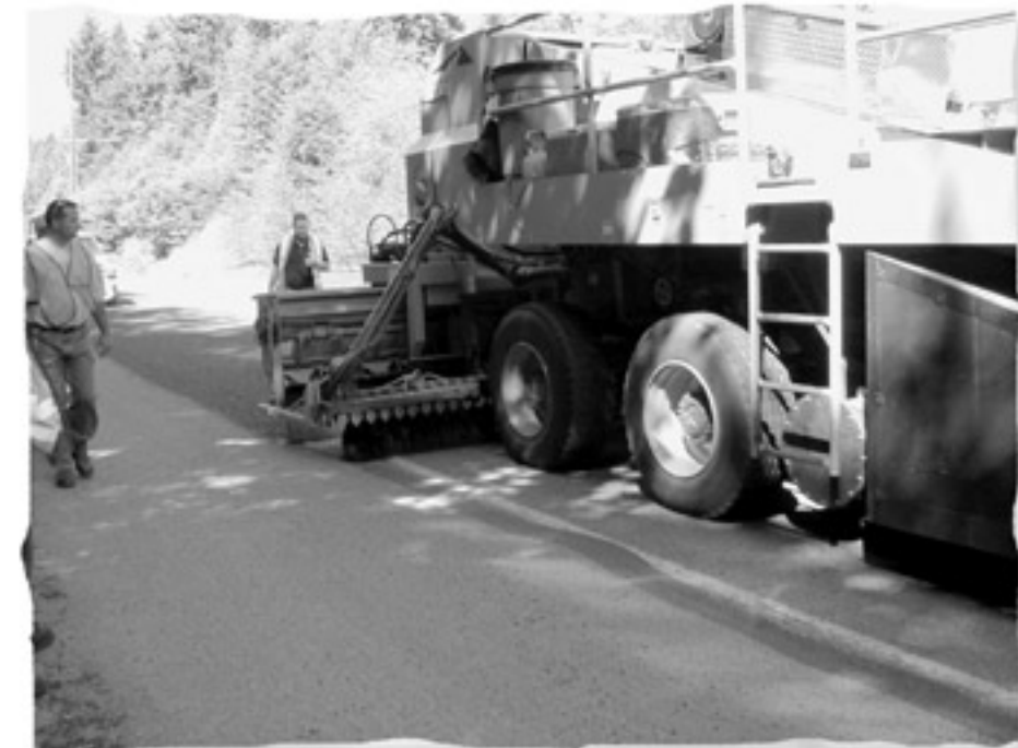
RoadArmor machine applying emulsion and cover rock.
