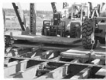
Garco Construction Corp. removing the old concrete bridge deck.
