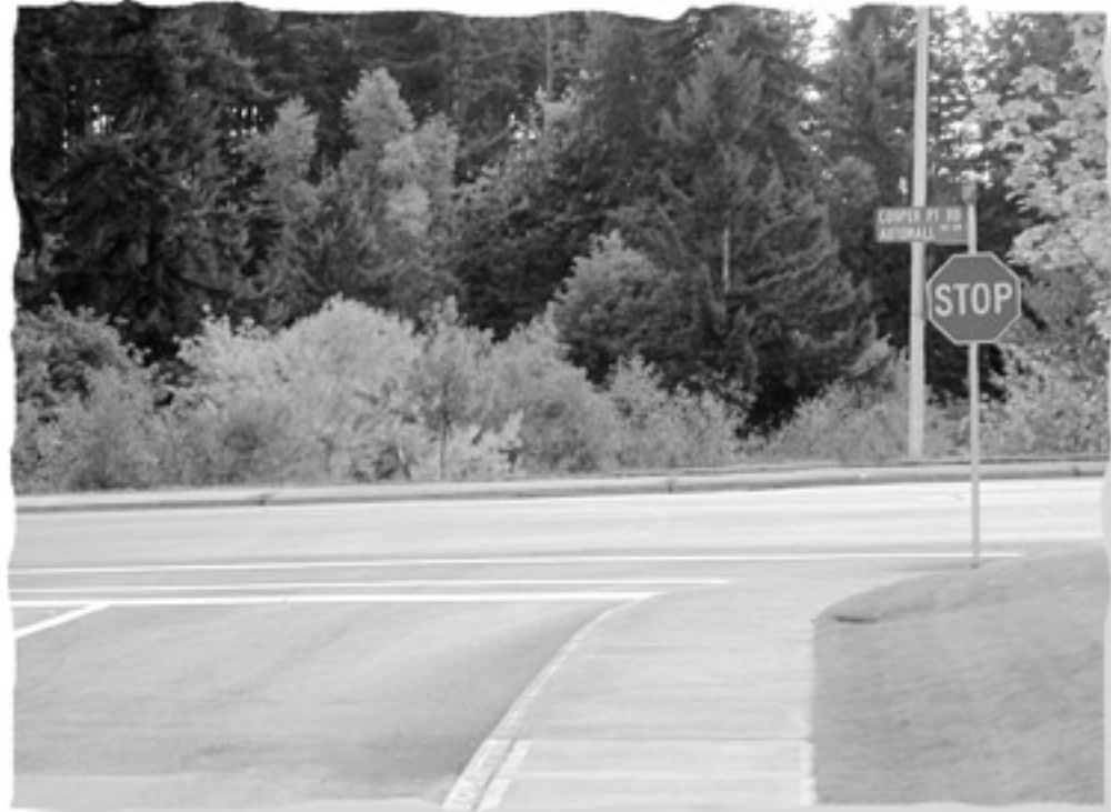
Figure 1. A properly installed STOP (R1-1) sign stop line, and crosswalk.
