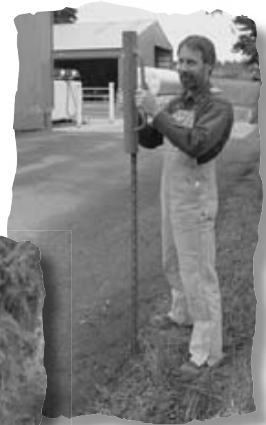
Driving T-post with standard T-post driver.
