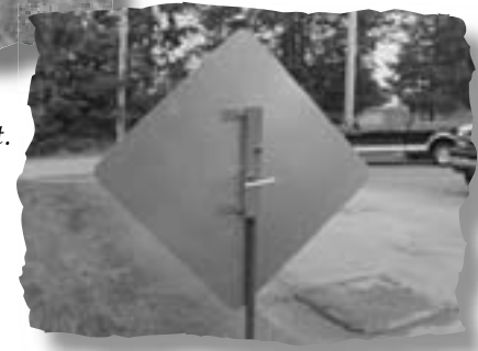
T-post adapter installation.
