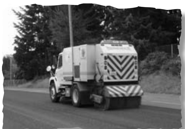
Sweeping the loose rock.
