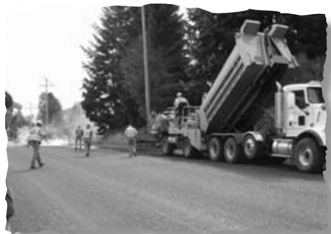
Spreading the pre-coated rock.
