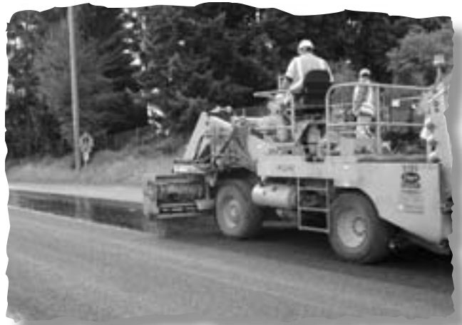
Spreading the pre-coated rock.
