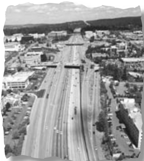
Photo 1 – Looking north up I-405. The overpass closest to the foreground is the old NE 4th Street bridge.
