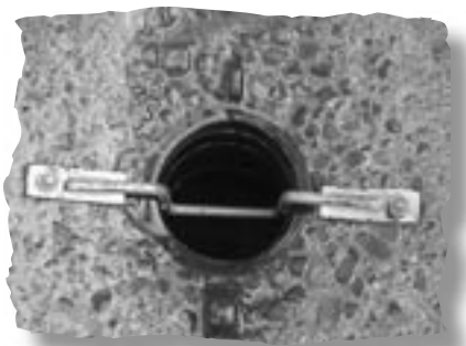
Restrictor rod device installed.
