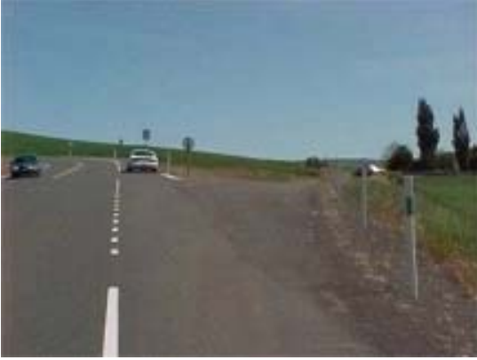
4 Johnson Hollow Road - sight distance problem MP 370.8
