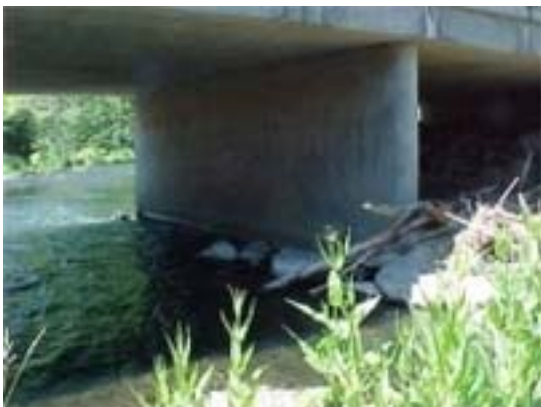
Touchet River Bridge – frequent scouring problems MP 361.49
