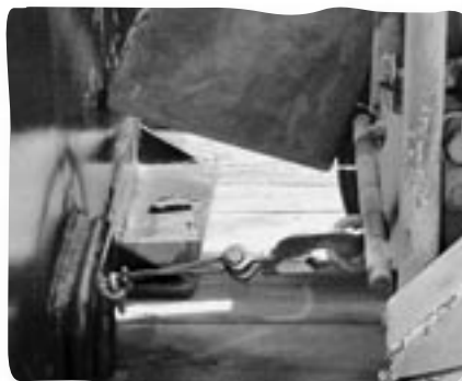
Hook and cable from wench for pulling the unit into place.
