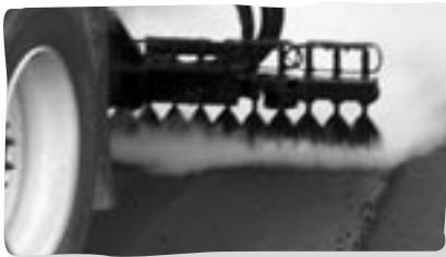
Image 7 — Proper overlap and spray bar height.
