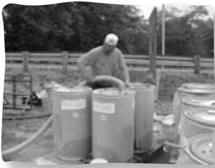
Loading Part A into Water trucks
