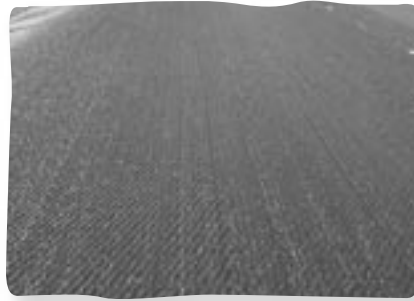
Image 9 — Proper coverage on a milled surface.
