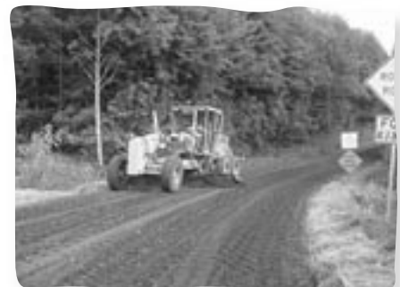
Grader shaping and blending
