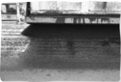
Image 5 — Excessive tack (unbroken).
