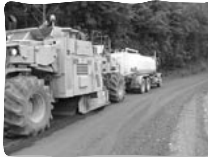
Mixing PX-300 into road base
