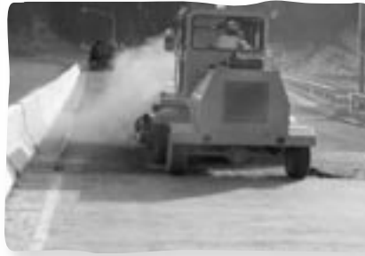
Image 1 — Brooming roadway surface.
