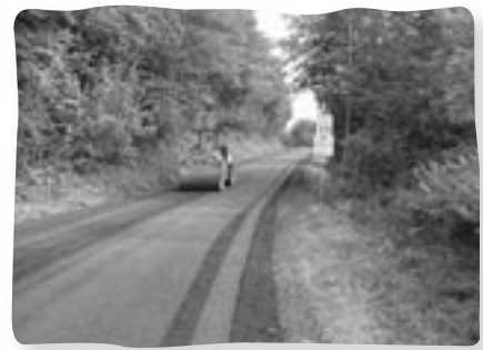
Final compaction using steel-wheeled roller
