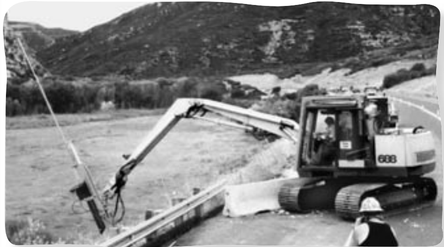
Soil Nail Launcher
