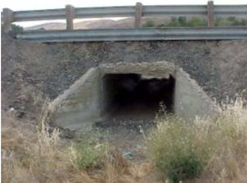
3 Improve culverts (MP 40.71 and MP 40.9)
