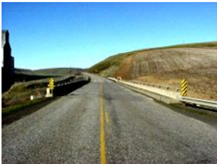
Harshaw Rd. Bridge # 124/014 MP 27.48
