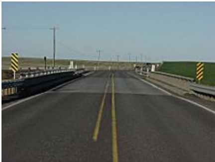
Old BN RR Bridge # 124/008 MP 22.62
