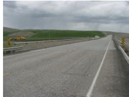
Winnett Cnyn Bridge 124/012 MP 25.16
