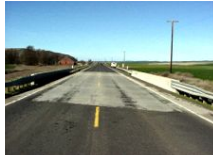
Whetstone Bridge # 124/020 MP 35.45
