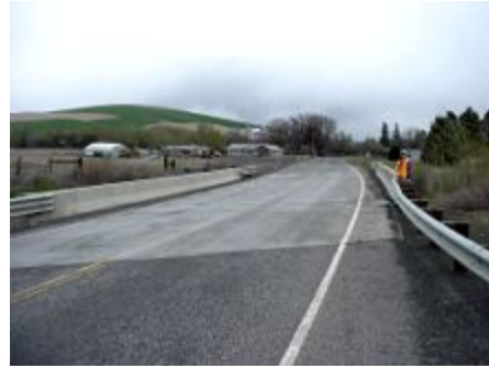
Coppei Creek Bridge # 124/028 MP 44.20
