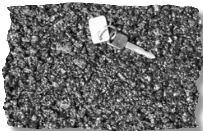
Photo 1 – NovaChip® asphalt placed as a surface treatment.
