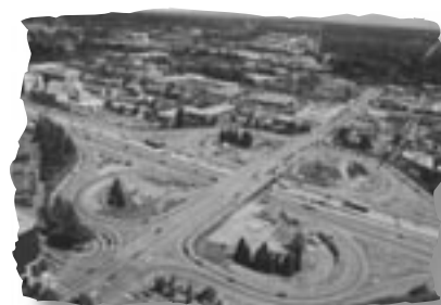
Summer 2002. The NE 8th interchange with the old bridge. Construction was beginning on the new south half.
