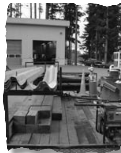
Guardrail sections and posts
