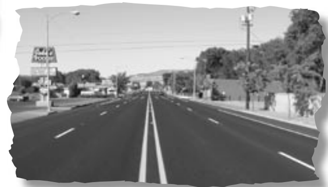
Photo 11 – Soap Lake’s NovaChip® overlay.
