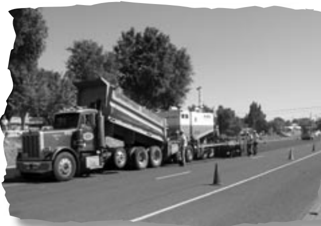
Photo 8 – Delivery of the NovaChip® asphalt to the Novapaver.
