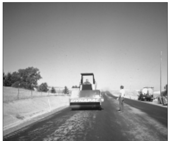
▲ Rolling the concrete treated base
