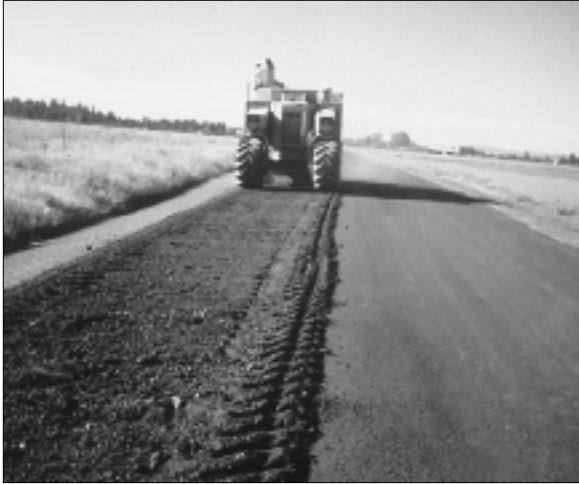
▲ CMI RS650 pulverizing the pavement
