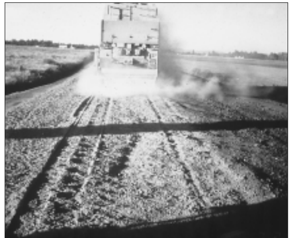
▲ Adding the concrete treated base
