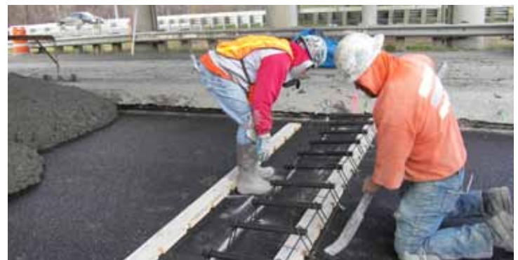
Crews install dowel bars to extend the life of the pavement.
