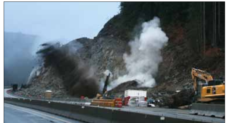
Controlled rock blasting will make room to widen I-90 to six lanes.
