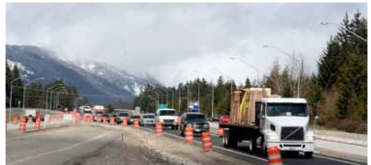
Crews reroute traffic through the work zone along I-90 near Easton.
