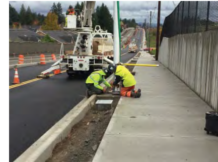
Vancouver: NE 18 th Street Construction
