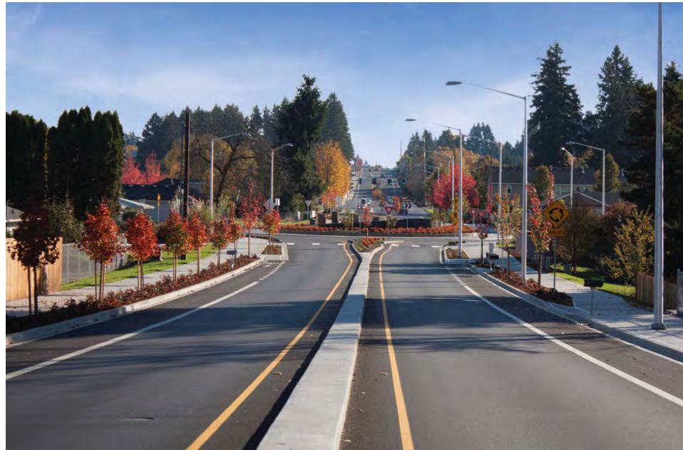
Vancouver: NE 137 th Avenue Roundabout
