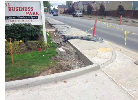
Clark County: NE 10 th Av. Construction
