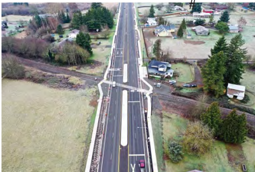
NE 119 th Street RR Crossing
