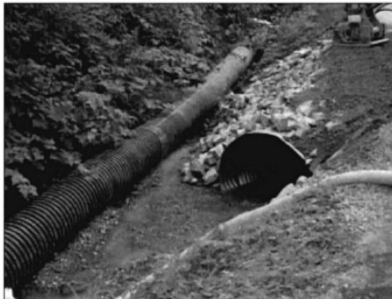
A stream bypass used to divert water around a construction site
