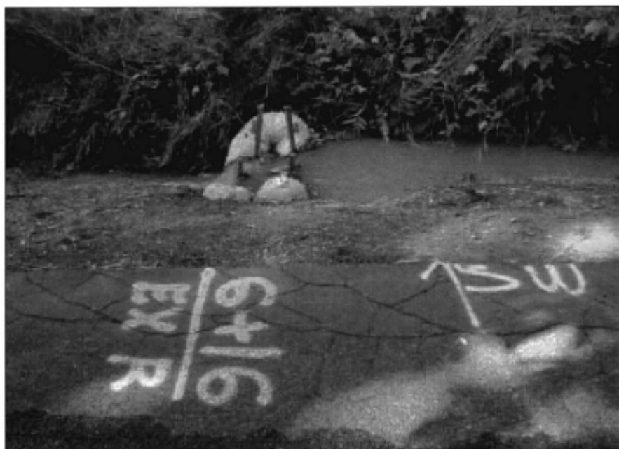
Coir log used to allow settling and to decrease water velocity/erosive forces
