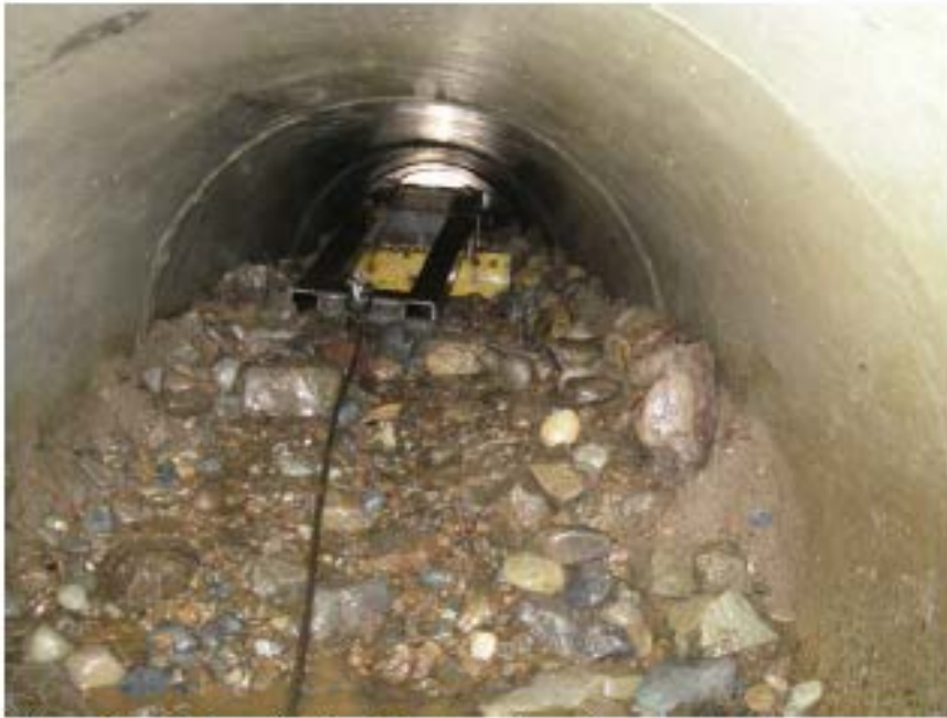
Figure 6: Pull Dozer in the culvert seen from the culvert outlet.
