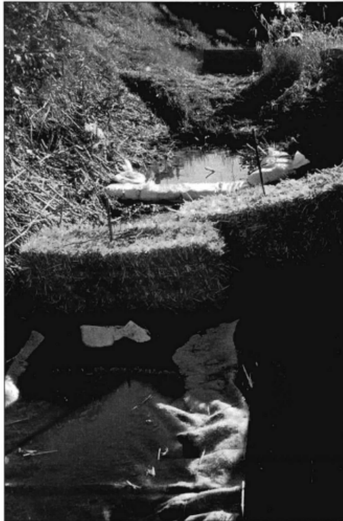
Straw Bale Barrier (2) reducing water velocity and erosive forces. Note other BMPs also being used
