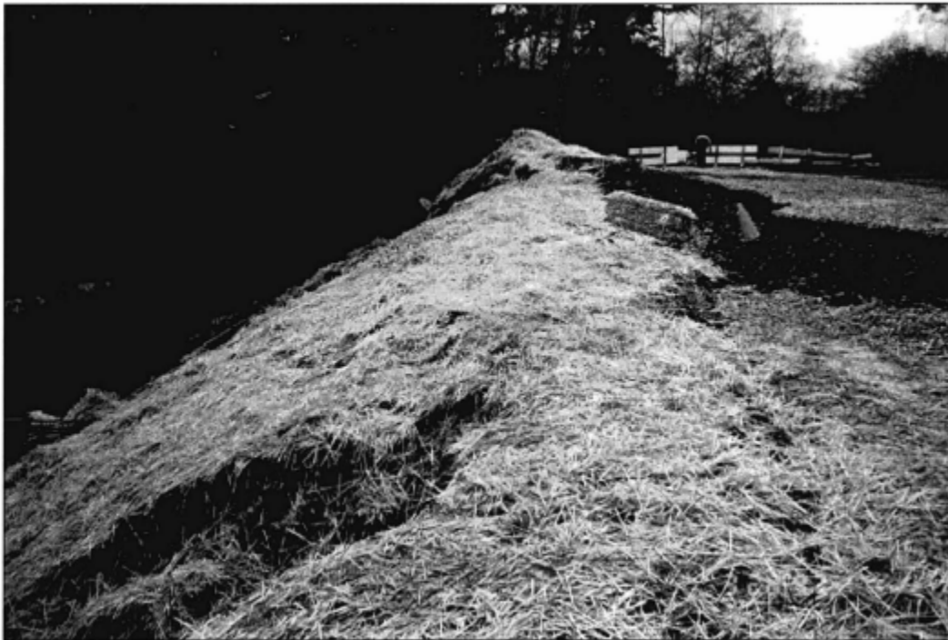
Using straw to reduce erosion in a slide area prior to a major stabilizing project
