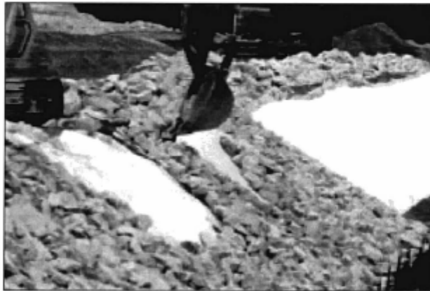
Rip rap placed on slope for increased stability
