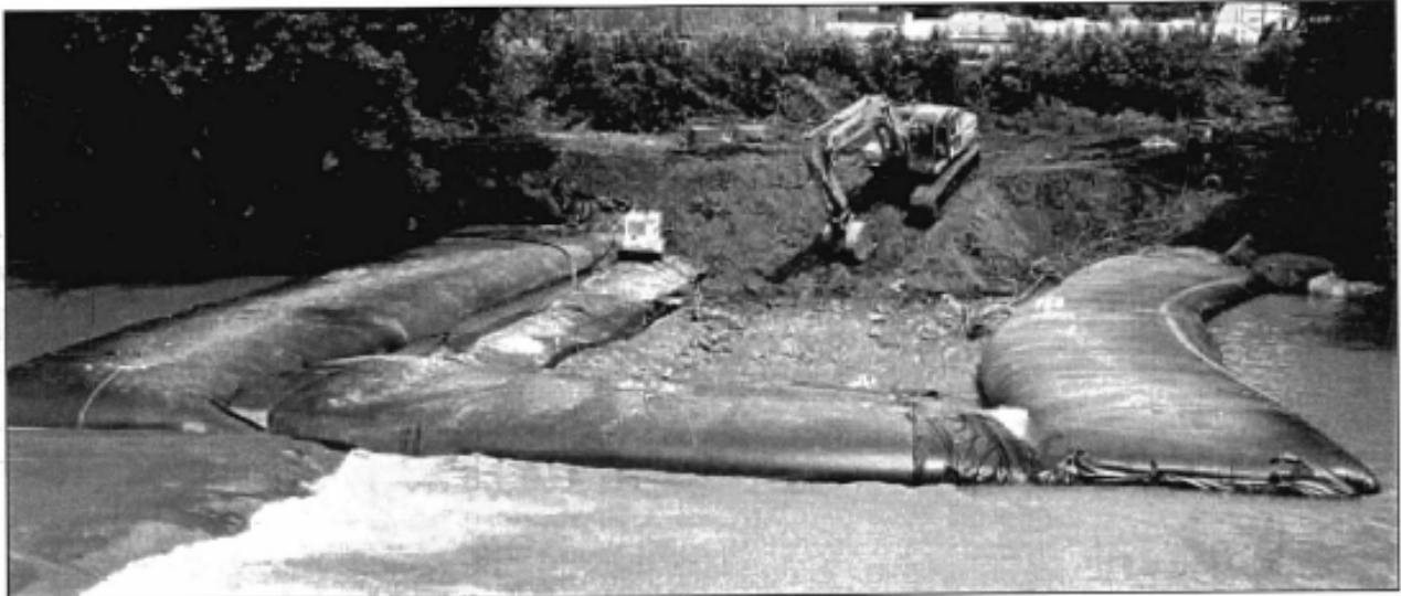
Aqua barrier used as coffer dam
