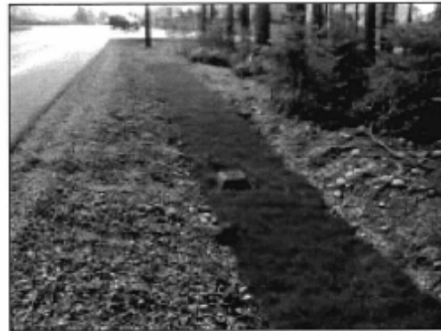
Grass lined channel: providing a filter
