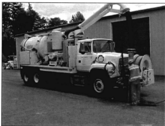
Vactor truck removing sediment from catch basin
