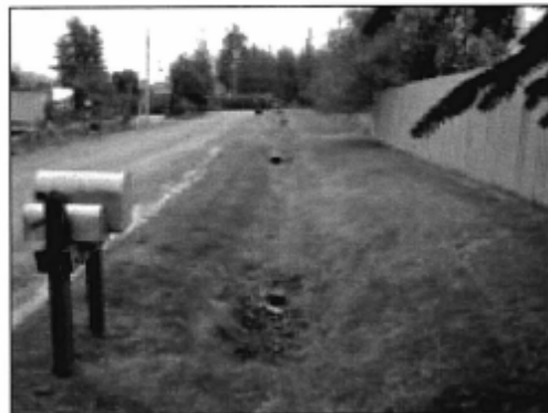
Grass lined channel: reducing erosion by providing ground cover
