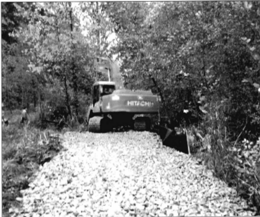
Access road installation
