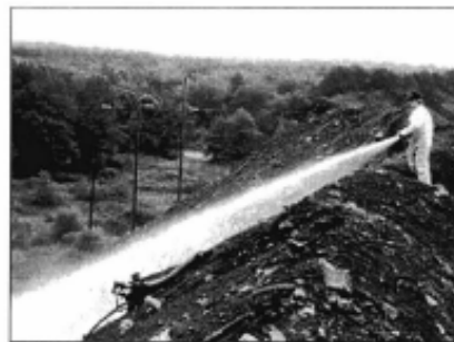
Wetting down stockpiles to reduce airborne soil particles
