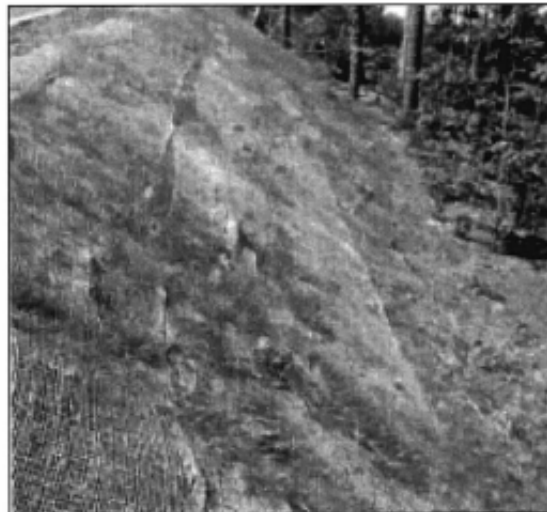
Stabilizing the soil using matting and hydroseeding
