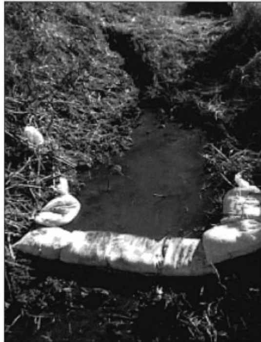
Sandbags filled with washed rock acting as a filter
