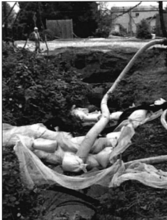
A stream bypass used to divert water around a construction site
