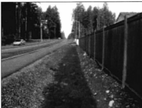
Grass lined channel: providing a filter
