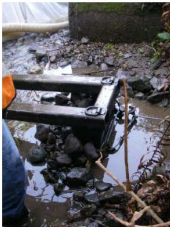
Figure 7: Pull Dozer with large cobbles removed from the culvert.
