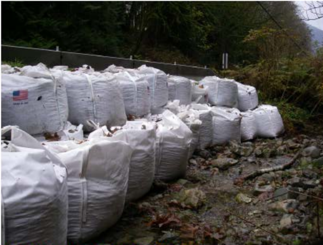
Figure 12 Temporary stream bank protection with Supersacks®.
