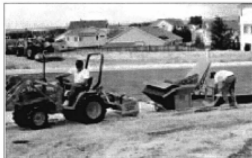
Continuous berm retaining soil particles and debris
