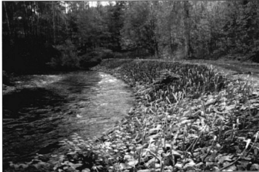
Staked streambank to provide vegetative cover once vegetation has established
