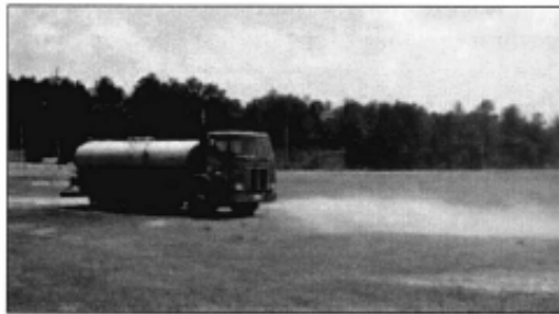
Water wagon wetting down field for dust control
