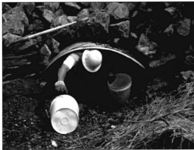
Placing streambed gravel inside a newly installed cross culvert to provide a natural substrate for fish
