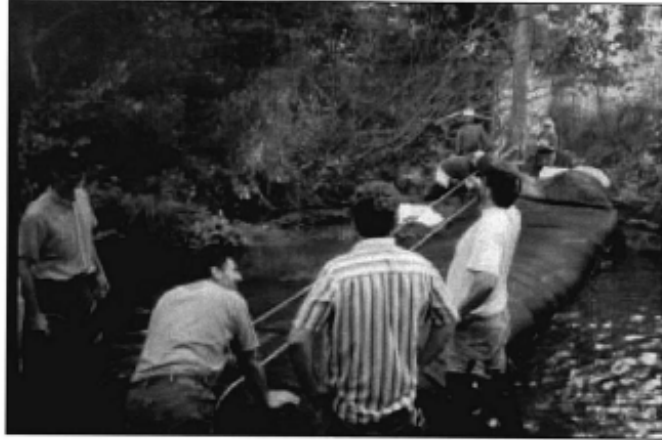
Installing aqua barrier in river to provide a dry construction area
