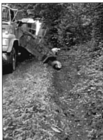
Using a ditchmaster to leave a vegetative buffer
