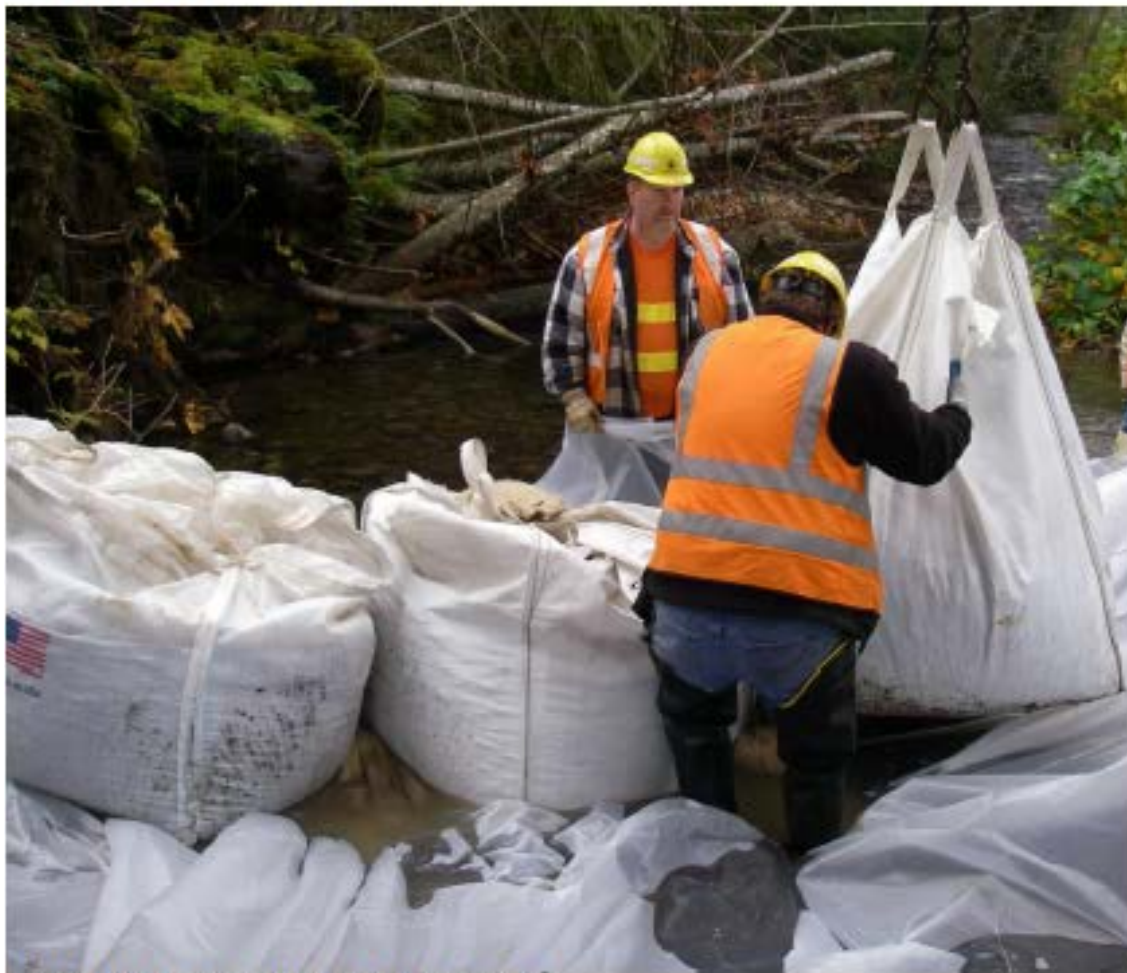
Figure 11 Building a coffer dam with Supersacks®.
