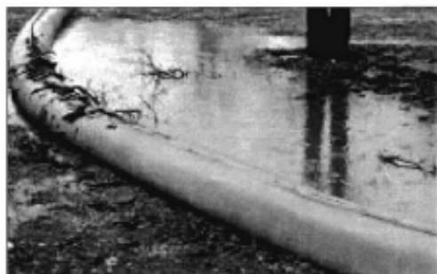
Continuous berm intercepting water from construction area
