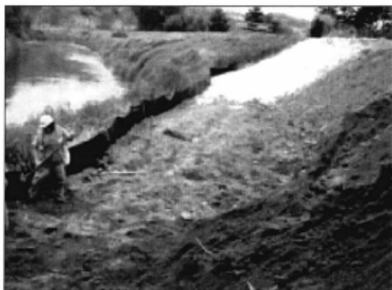
Silt fence being installed on a temporary access road; used as perimeter protection
