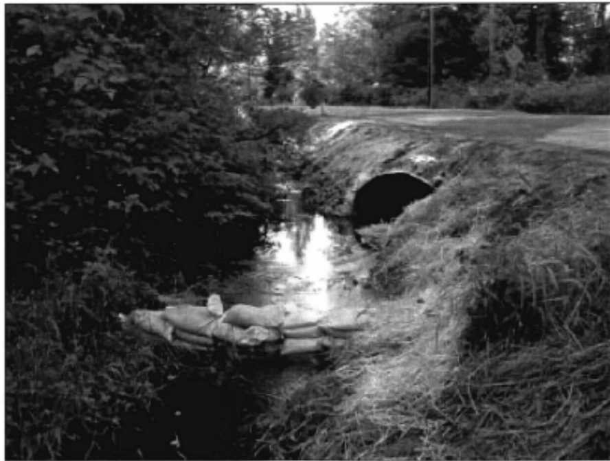
Sandbags used as a cofferdam
