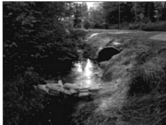
Sandbags acting as a barrier
