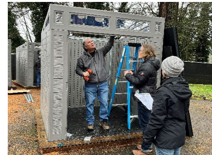
Vancouver Safe Stay Community tiny home building work party
