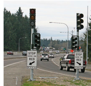
Ramp metering on I-5
