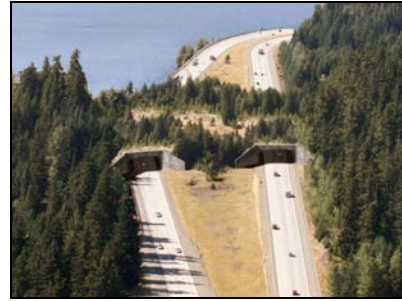
Within the project area, ecological connectivity structures would reduce wildlife/vehicle collisions.
