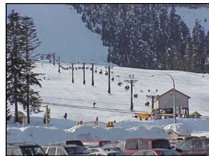
The I-90 project is just east of the ski area at Snoqualmie Summit (Shown: Summit West Ski Area)
