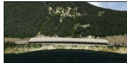
The new snowshed will cover the entire width of I-90, preventing avalanches from reaching the highway at this location. (Design Visualization)
