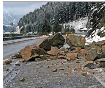
WSDOT regularly cleans landslide debris from I-90 in the project area.
