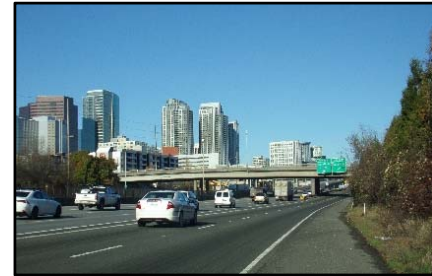
Existing Main Street Overpass
