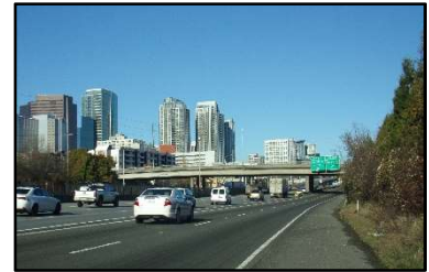
Existing Main Street Overpass
