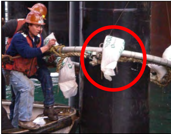
The red circle shows the sandbags strapped on to the metal rings for weight for bubble curtain one. Rope was strapped to the base of the bottom ring to cover the lugs and keep the ring flush with the seafloor bottom.
