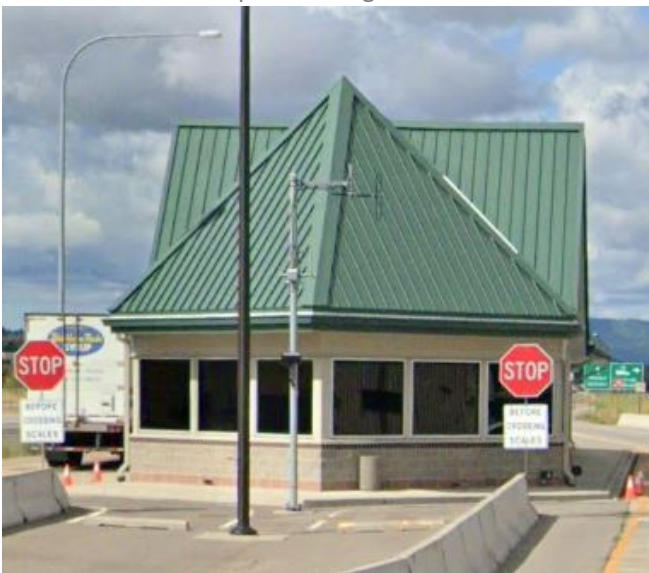
Exhibit 3-5: WSDOT Spokane weigh station scale house
