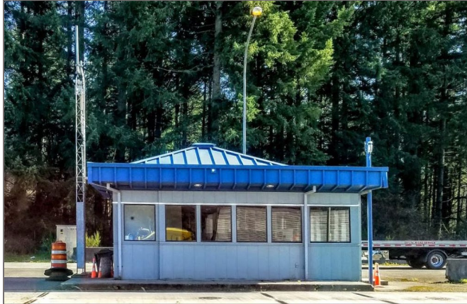
Exhibit 3-1: Fort Lewis Weigh Station Scale House 7
