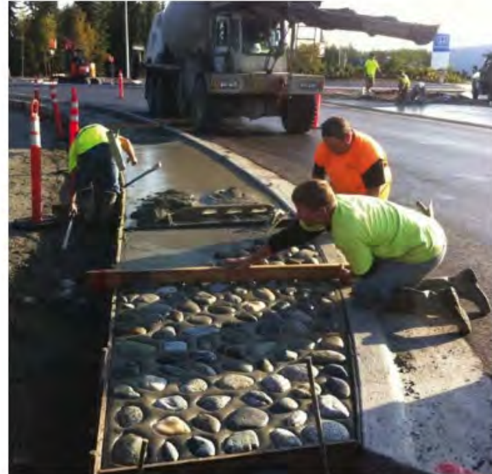
Exhibit 14.16. Example of embedded river rock being placed in the buffer.
