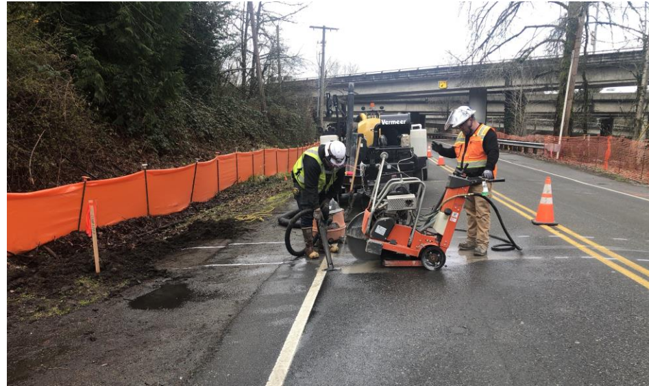
Crews performing saw cutting work on Woodinville Dr.
