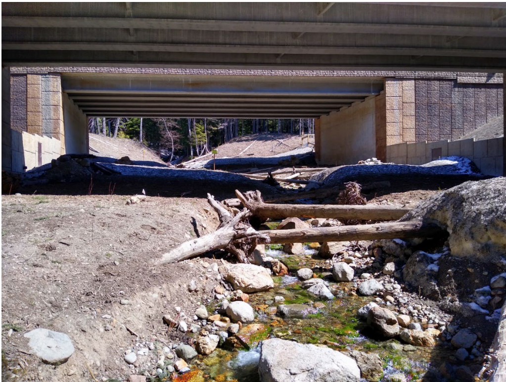
Wildlife bench example at a large structure.
