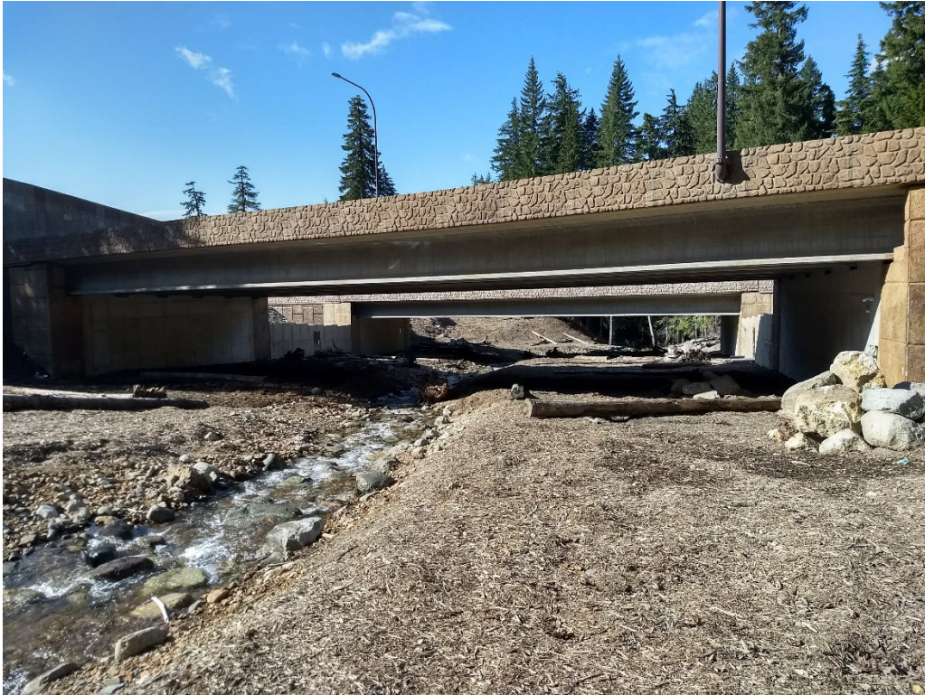
Wildlife bench example at a large structure.
