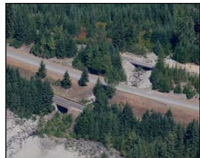
USFS bridge upstream of I-90 at Rocky Run Creek.
