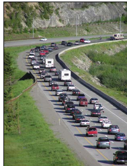
Traffic volumes over Snoqualmie Pass often exceed the design capacity of the highway.
