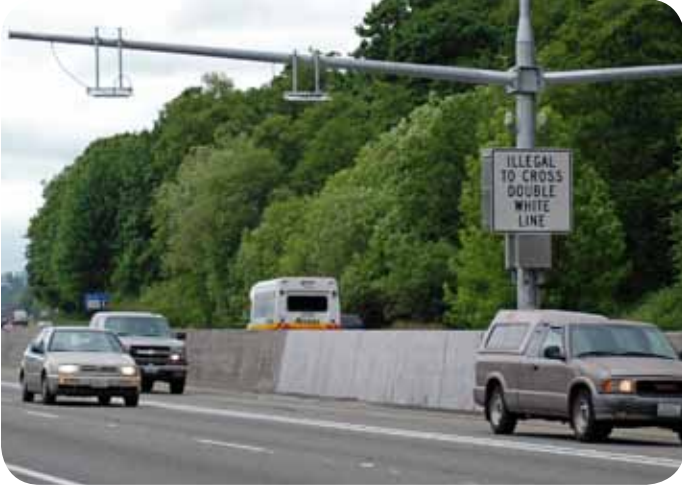
The antenna for electronic tolling on SR 167 HOT lanes
