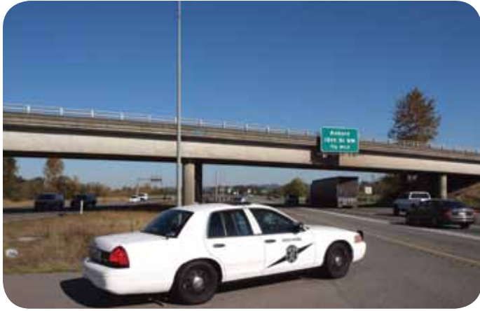
The Washington State Patrol provides additional enforcement on SR 167. HOT lanes compliance is estimated to be 95–97 percent.
