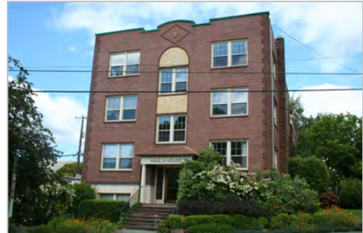
Hamlin House – 222 East Hamlin Street
