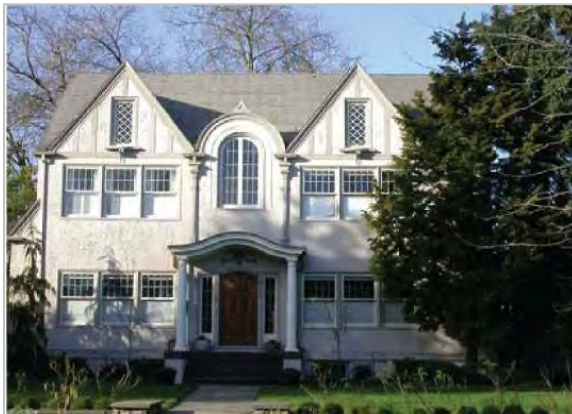
Exhibit 5-21. 2158 East Shelby Street, Montlake Historic District
