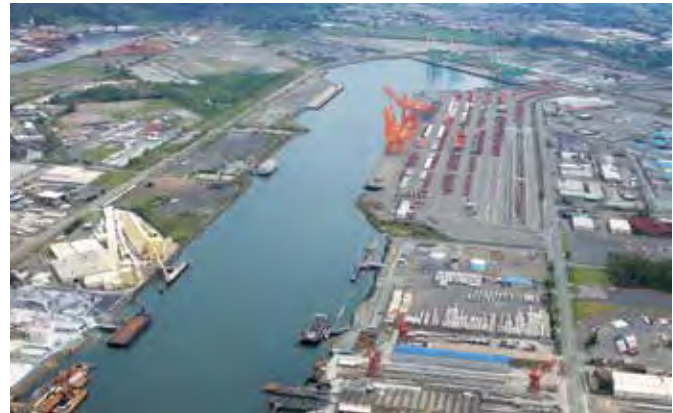
Relieves traffic congestion and completes a critical freight link between the ports of Tacoma and Seattle.
