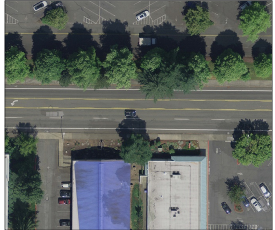
Roadway Resurfacing Road Diet After Capital Mall Blvd, Olympia WA
