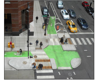
Protected Intersection Source: NATCO
