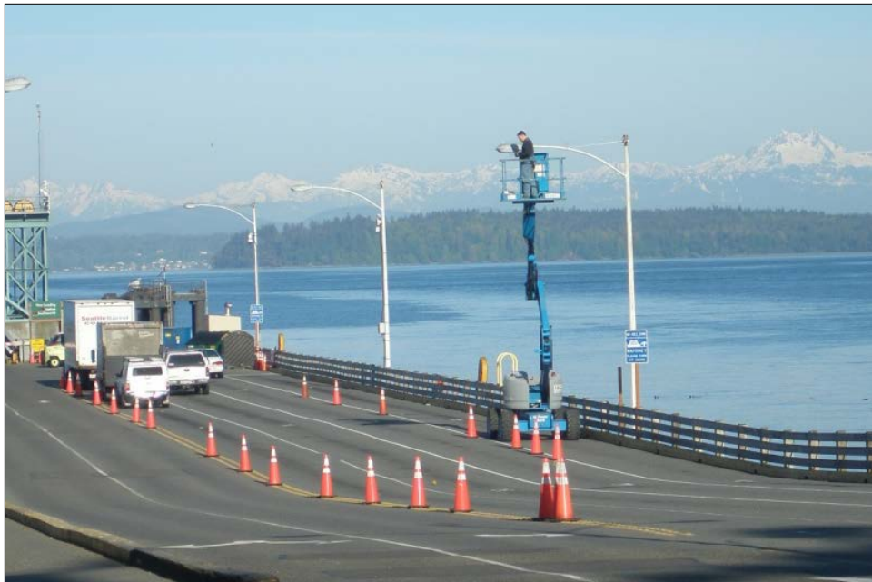
Manlift in Use at WSF Terminal Exhibit 440-10
