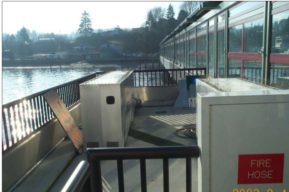
Clinton Ferry Terminal Backflow Preventer Enclosures Exhibit 440-18
