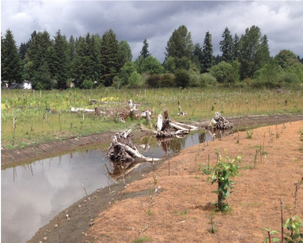
Figure 10A-2 Rootwad Habitat Structures, Evans Creek, King County
