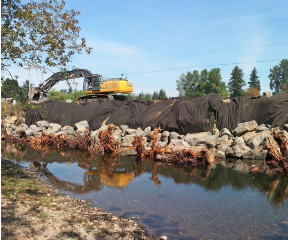
Figure 10A-3 Log and Rock Revetments, Newaukum River, Lewis County
