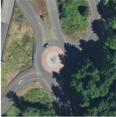
Roundabout showing two-color mountable central island. Location is State Route 432 at Exit 36 on Interstate 5 in Kelso, WA
