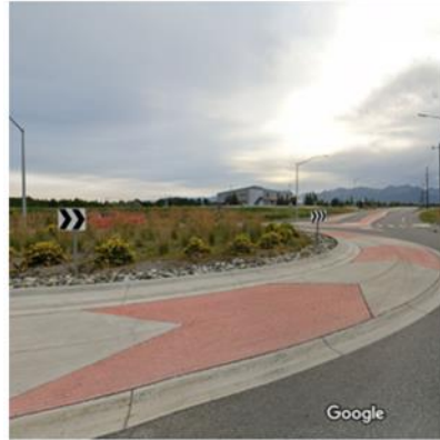
Roundabout apron with a chevron pattern at West 100th Ave and Northbound ramp terminal at the Walter J. Hickel Parkway, Anchorage, AK
