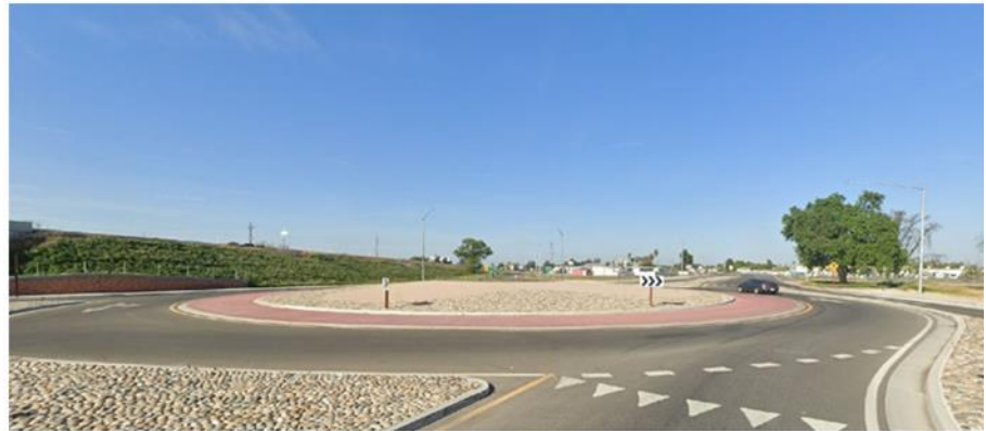
Roundabout that provides range of textures, colors, and shapes to achieve contrast. This example includes a rock blanket on the splitter islands, sidewalk buffer, and a wave pattern on the central island. Contrasting the rock blanket in the central island is tan concrete with brick texturing. Further contrast is provided by the red brushed concrete apron and a small circular landscaped area in the central island. The truck apron is red brushed concrete. The rock blanket could be placed in pervious concrete if needed for stormwater management purposes. Location is Handford Armona Rd at Exit 84 on State Route 198 in Handford, CA.
