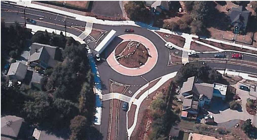
Single lane roundabout - Truck using the truck apron
