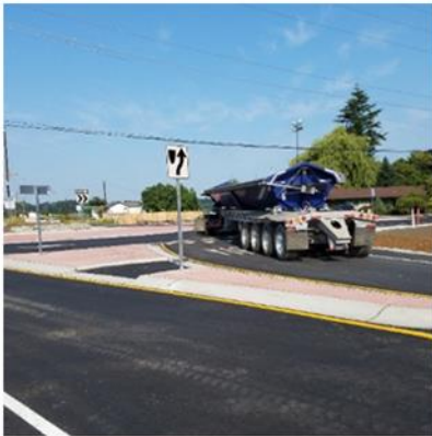
Roundabout showing red concrete with brick texturing for the splitter island and central island, landscaped central island, and gravel and natural plantings at the edge of pavement. Location is State Route 9 at Francis Rd in Skagit County, WA
