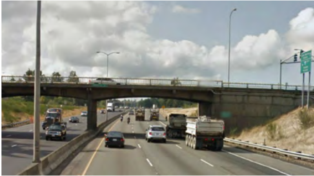
Figure 13 Many of the existing bridges crossing I-5 in the study area limit the ability to widen the freeway, such as this one at the Berkeley Street interchange.
