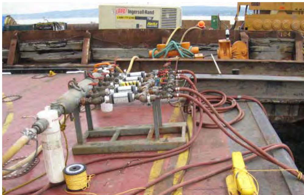
Figure 8: Photograph of the bubble curtain being deployed
