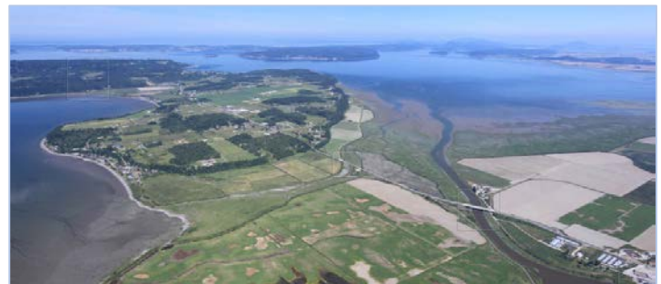
SR 532 Camano Gateway and Davis Slough Bridge
