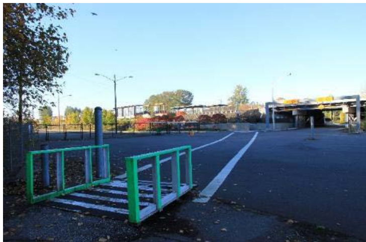
ADA ramp and striping.
