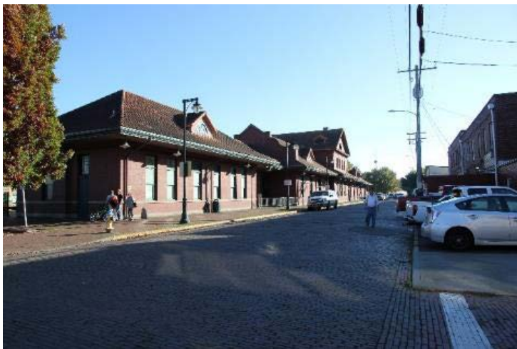
Centralia Station frontage to Railroad Ave.
