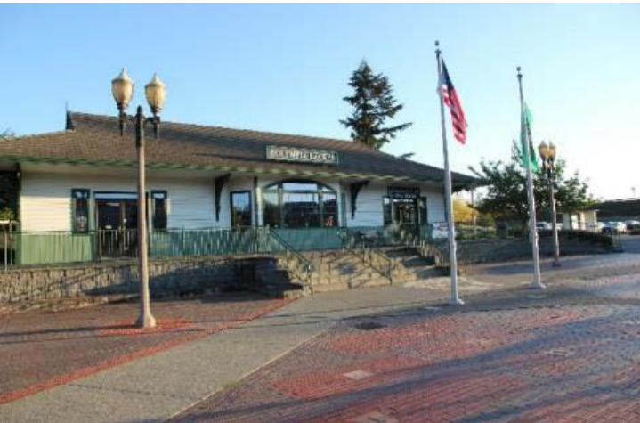
Olympia-Lacey Station exterior.
