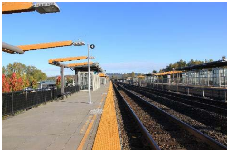
Tukwila Station platform and RR tracks.
