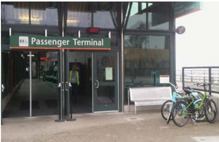
Entrance to the Ferry Terminal.
