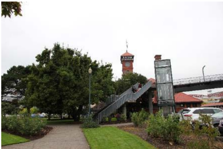
Pedestrian grade-separated crossing over station platforms.
