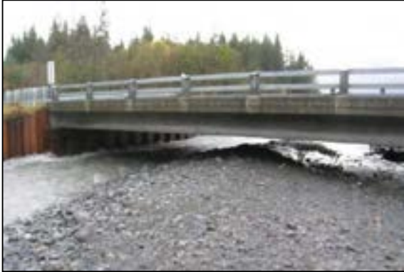
Figure 150. Bridge elevation view of channel condition. (Source: Alaska DOT)
