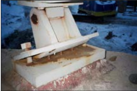
Figure 145. Misaligned rocker bearing. (Source: Alaska DOT)
