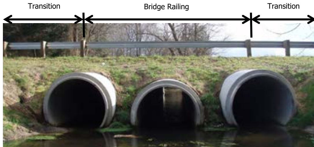
Figure 12. Metal bridge railing and transition for long-span application. (Source: Delaware DOT)
