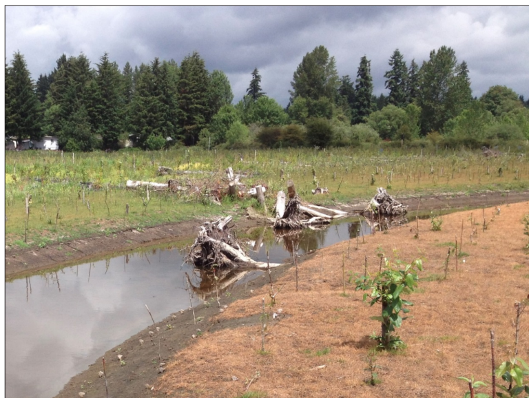
Figure 10B-2 Rootwad Habitat Structures, Evans Creek, King County
