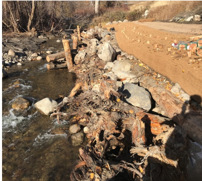
Figure 10B-5 Crib Wall with Steel Piles, Sauk River Side Channel
