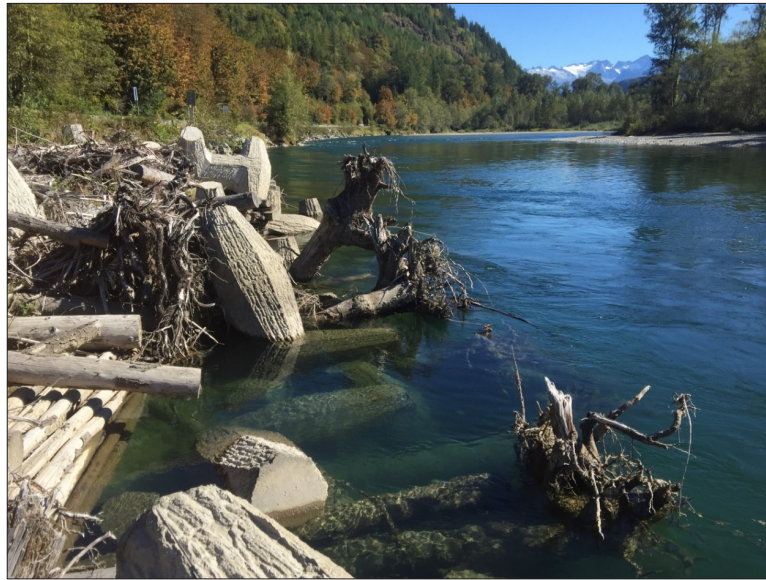
Figure 10B-8 Dolotimber Structures, Skagit River
