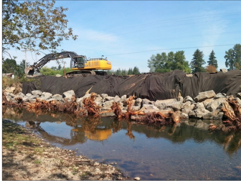
Figure 10B-3 Wood Studded Revetments, Newaukum River, Lewis County
