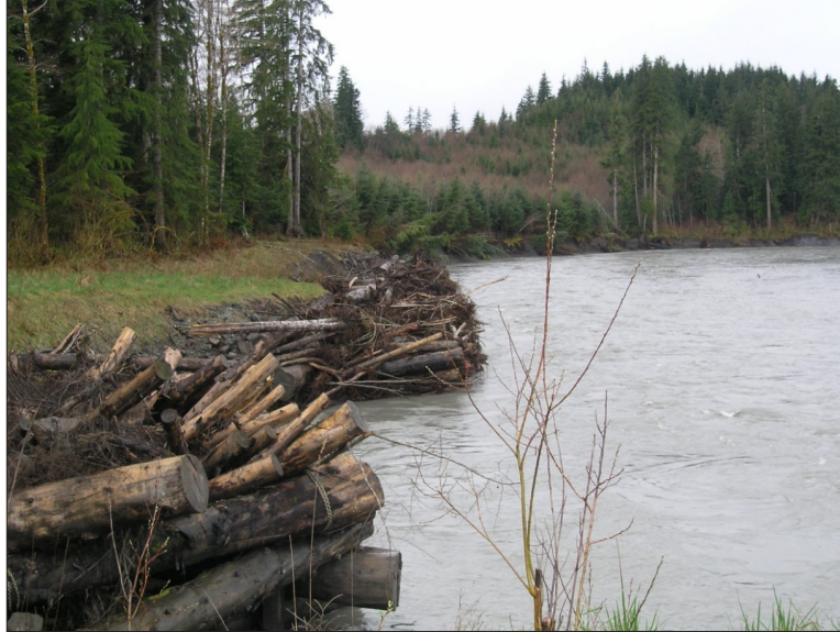
Figure 10B-6 Flow Deflection Jams, Hoh River, 2004
