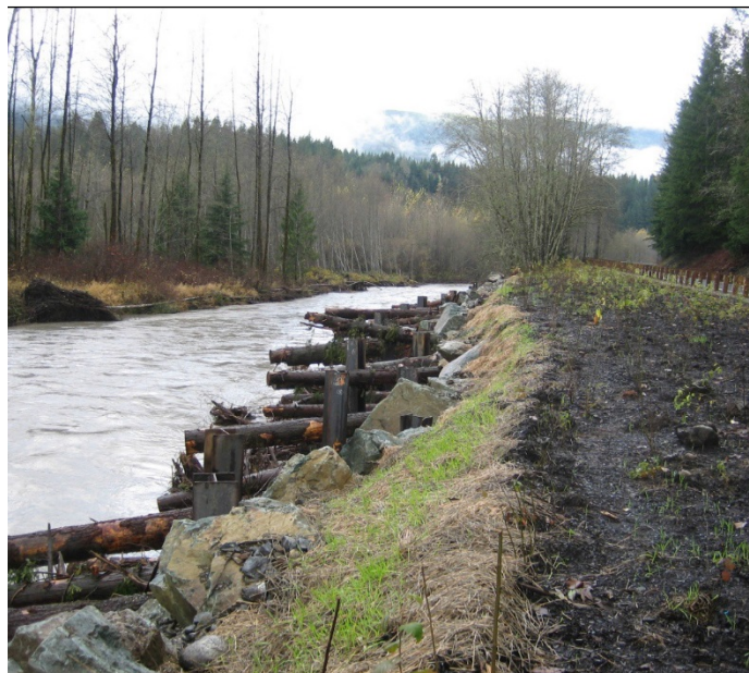
Figure 10B-5 Crib Wall with Steel Piles, Sauk River Side Channel
