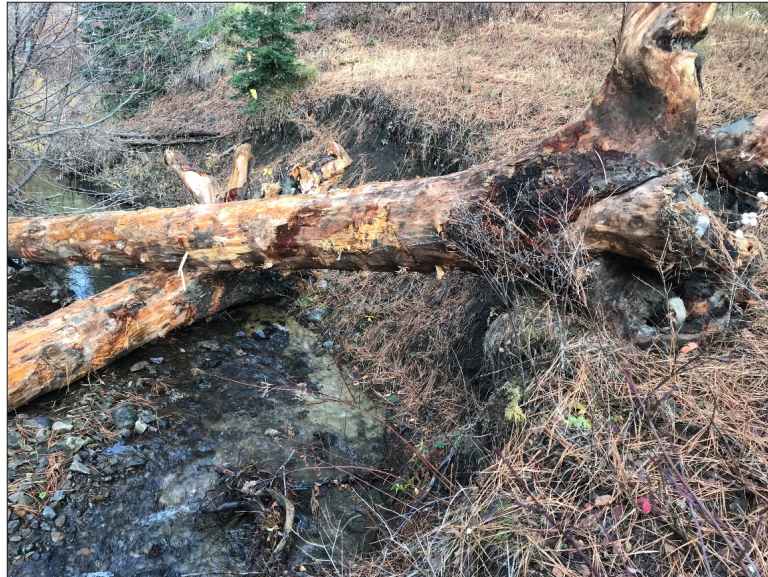
Figure 10B-1 Self-ballasting Large Wood Structure, Swauk Creek, Kittitas County
