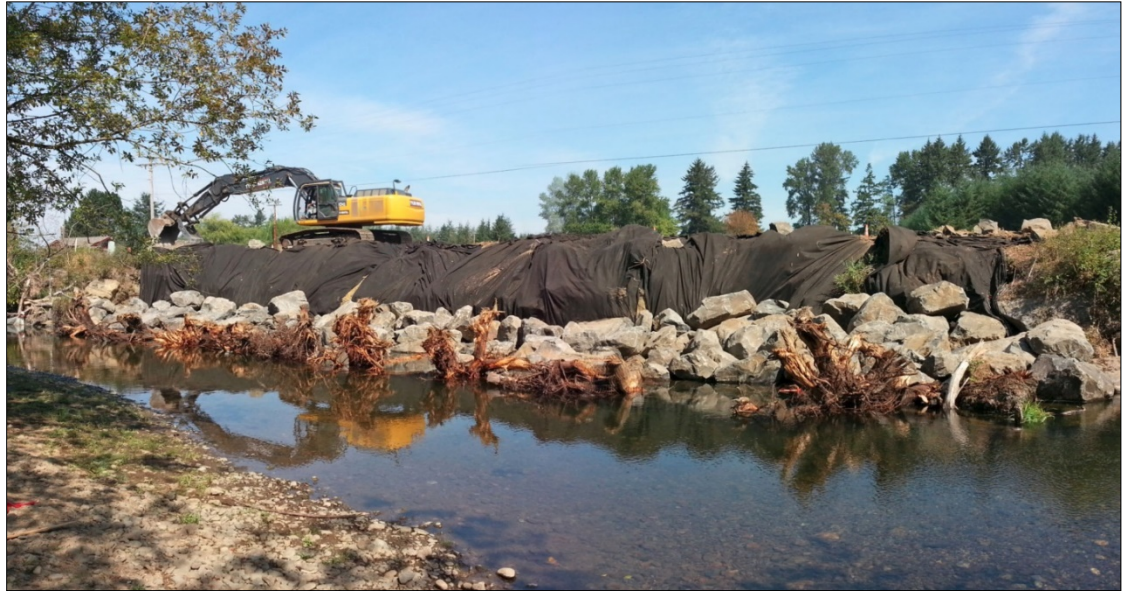
Wood studded revetments Figure A-2
