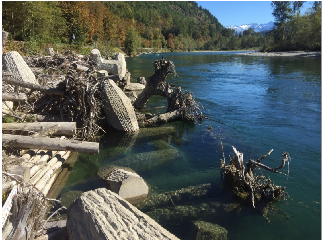
Dolotimber structures Figure A-6
