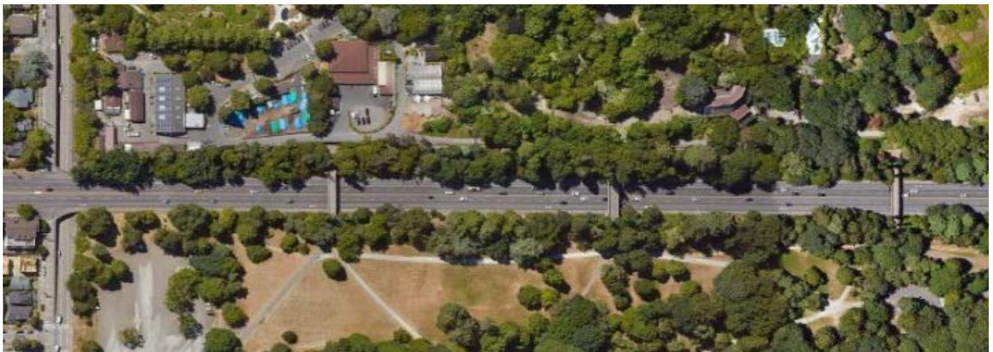
Figure 3-31: Three WSDOT-owned pedestrian crossings, spaced about 600 feet apart, are found between Woodland Park and the Woodland Park Zoo in Seattle.
