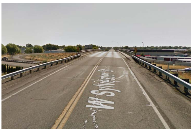
Figure F-22: Bridge gap in Pasco not identified through network analysis approach to finding network gaps. Bridge 395/102 on West Sylvester Street passes over SR 395. SR 395 at this location is prohibited to pedestrians and bicyclists, so it was not identified as an active travel gap. Bridges associated with active travel gaps were identified, but the presence of such gaps was only evaluated on the state highway system. This bridge, which connects residential and commercial areas of Pasco, has a narrow sidewalk on one side and no shoulders and therefore presents a local system barrier for pedestrians and bicyclists. The city has expressed interest in improving active transportation connections here.
