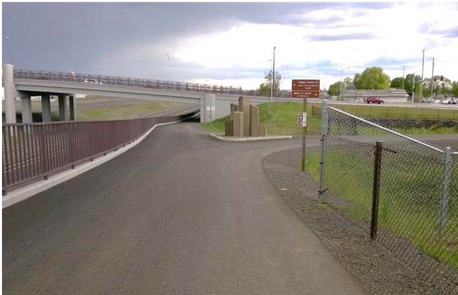
Figure 3-28: The Children of the Sun Trail in north Spokane along State Route 395, constructed as part of a Connecting Washington project. Source: TrailLink.
