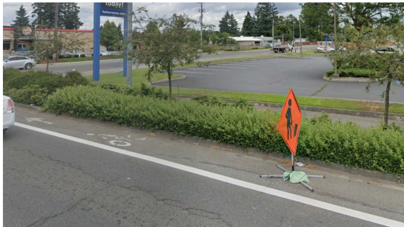
Figure 6-1: An example of work zone sign placement that violates the MUTCD. Image from Google Maps.
