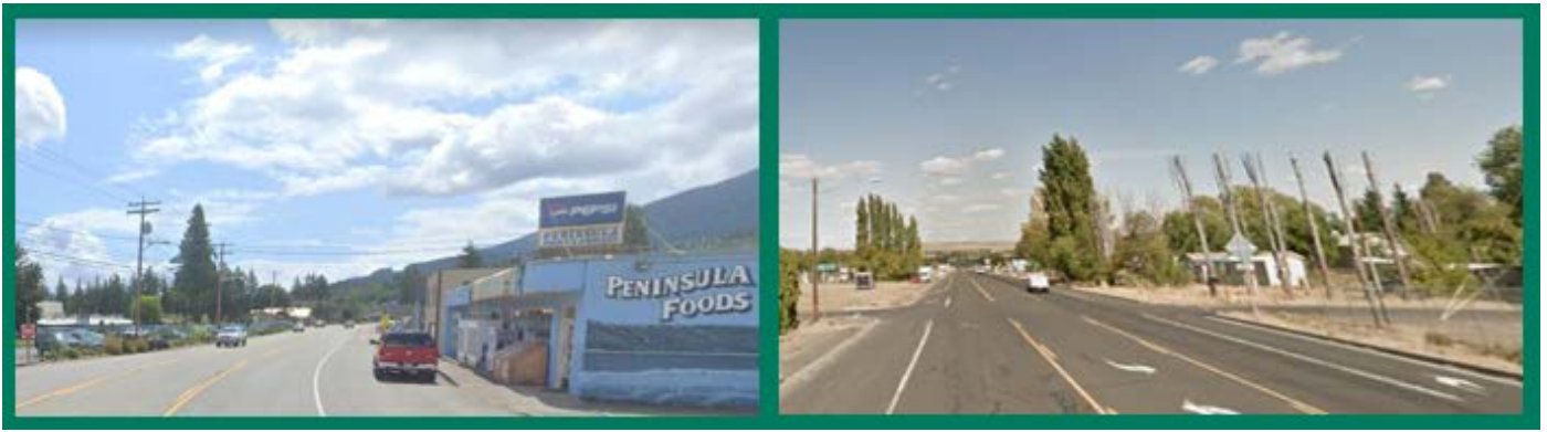
Figure 4-7: Posting a lower speed limit is only a partial solution for achieving a lower speed. Roadway characteristics need to change as well. It may be more costly to design for a lower operating speed when the roadway at the intersection is functioning at 50 mph with five lanes (Lakeview, right image) than on a roadway at an intersection that is posted at 30 mph with three lanes (Quilcene, left image). Image source: Google.
