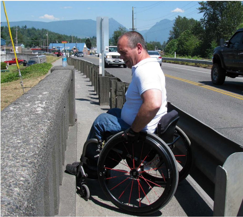
Figure B-1: As described in grant applications, this bridge over the Sultan River on U.S. 2 illustrates the kinds of gaps found on the state system: “The purpose of the Project is to construct a new bridge to provide safe passage for pedestrians and non-motorized users such as bicycles and wheelchairs across the Sultan River. Currently, the only pedestrian and bicycle connection between downtown Sultan and the portion of Sultan that is west of the Sultan River is an undersized pedestrian walkway on the north side of the existing U.S. 2 Bridge. The existing pedestrian and bicycle path is unsafe and does not meet Americans with Disabilities Act (ADA) requirements, including wheelchair accessibility. Both west and east-bound pedestrians and bicycles must share the same narrow path. The path also has a minimal separation between users and highway traffic.” City of Sultan is now building a new bridge to carry pedestrians, bicyclists, and utility connections.
