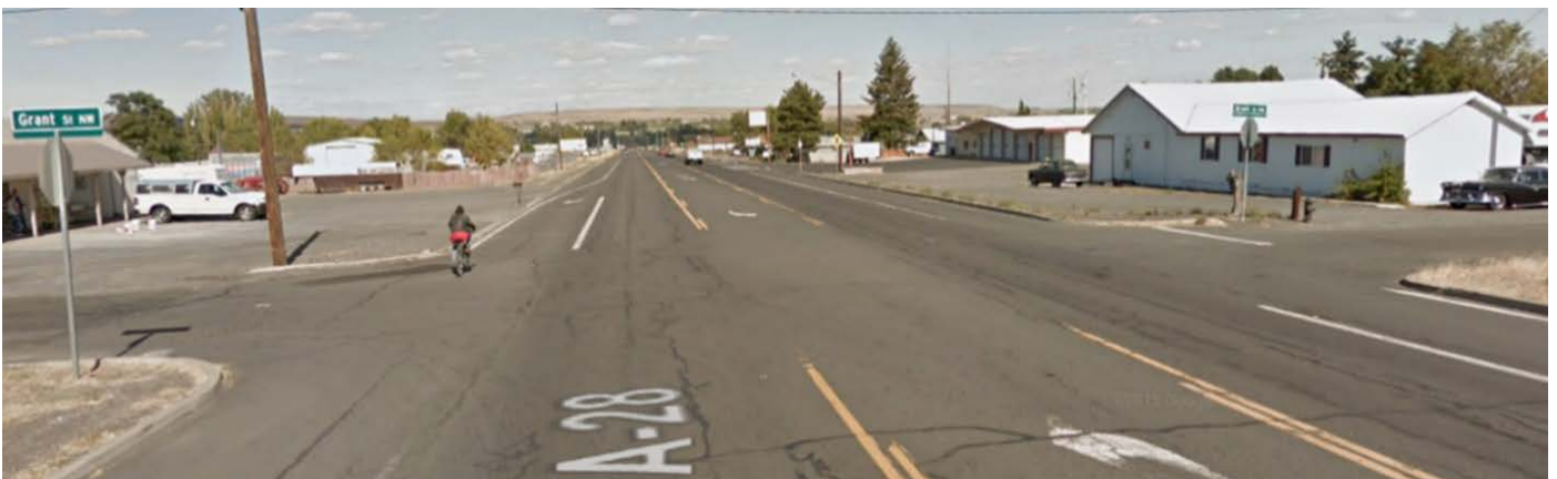
Figure 3-13: Intersection gaps. This image shows an intersection gap on State Route 28. The speed limit here is 50 mph on a stretch of highway with residences on both sides. People biking or walking must use what available shoulder exists. In this case, what appears to be a shoulder the bicycle rider is using is actually a right-hand turn lane. Here we also see the rider facing traffic. People riding bicycles may act in ways that feel safe to them; in this situation, the rider might be concerned about crossing high-speed traffic lanes to ride on the other side. Acting more like a pedestrian who is advised to walk against traffic, this person may feel this option is safer. Image source: Google Maps.
