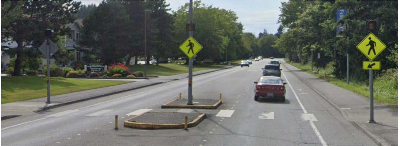
Figure 3-37: Enhanced crossing serving transit stops. This crossing of SR 11 in Bellingham provides a safe crossing opportunity for people accessing the transit stops on either side or other destinations nearby.
