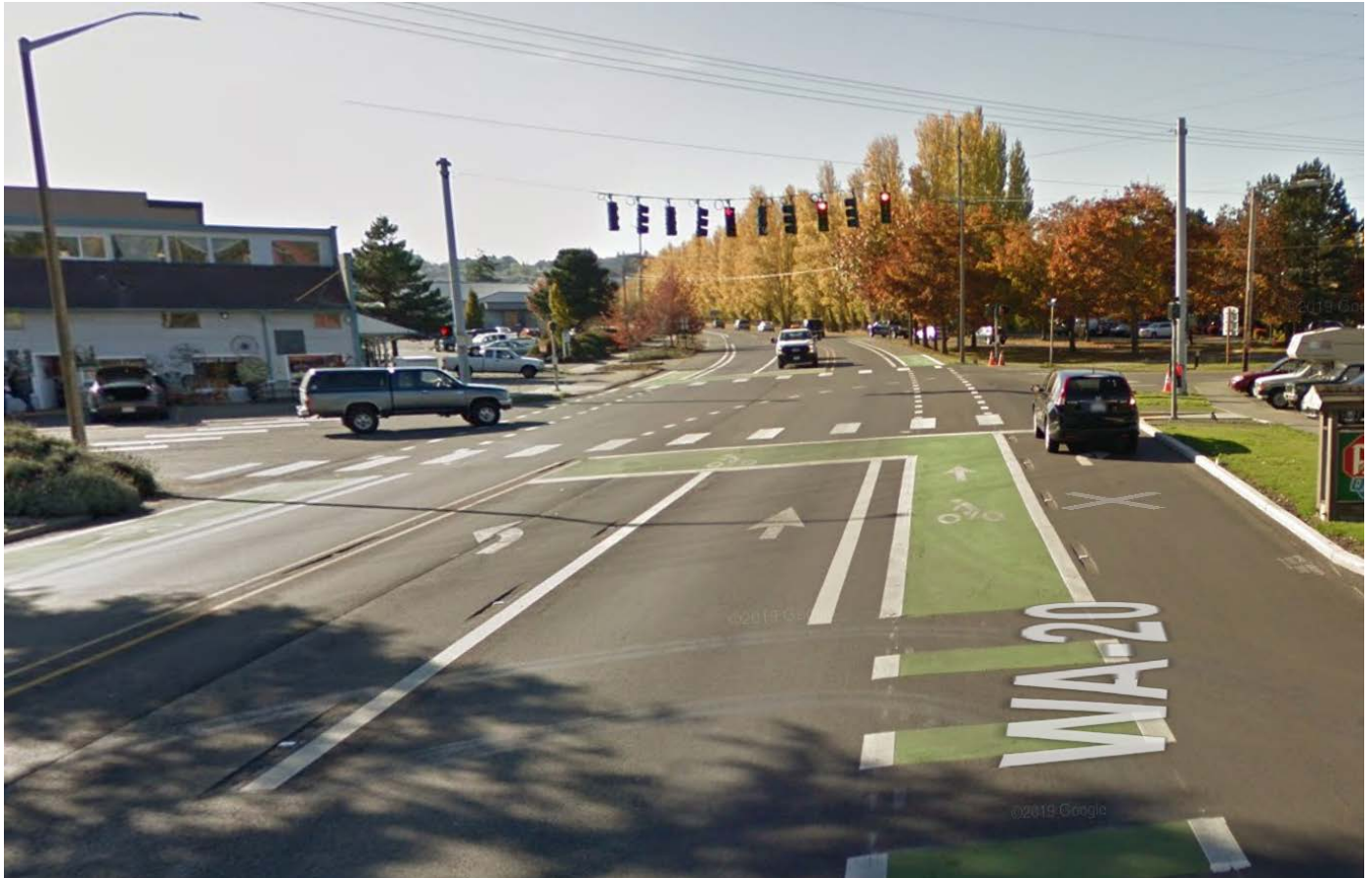
Figure F-18: Green painted bike boxes and bicycle intersection crossing pavement markings on SR 20 in Port Townsend. The wider dashed green markings in the foreground indicate to drivers that they are crossing a dedicated bike lane. The shorter dashed markings indicate that a bicyclist can be expected to proceed through the intersection.
