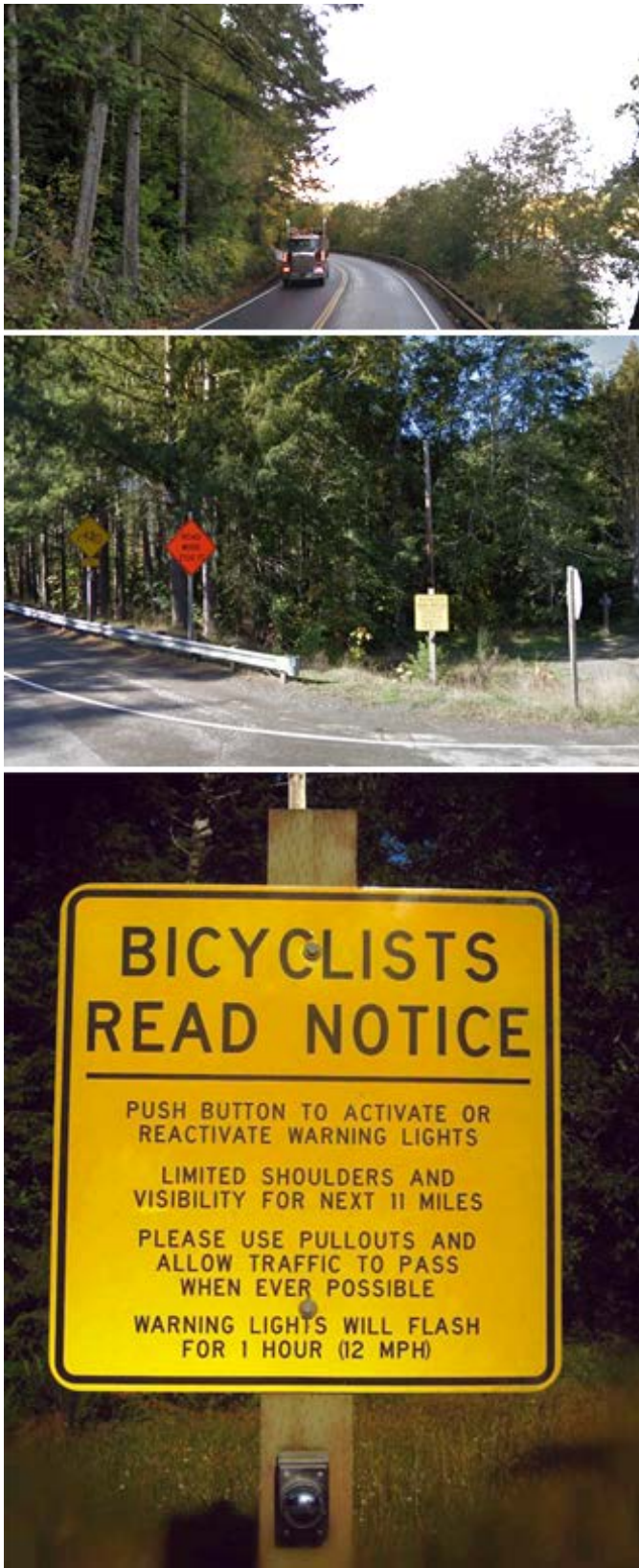
Figure 4-20: SR 101 along Lake Crescent where shoulders are not available and logging truck activity is relatively high. The posted speed on this section of highway has been reduced to 35 mph due to roadway space constraints. User-activated warning beacons are provided for bicyclists to alert drivers to their presence on the route, however the button may not be accessible to all users. The flashing signal will remain on for one hour, which is long enough for a person pedaling at 12 mph to pass through the area.
