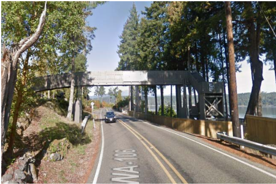
Figure 3-30: Pedestrian bridge near Union.
